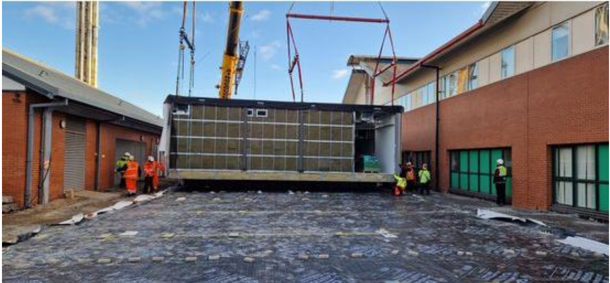
Site photo showing membrane installation
