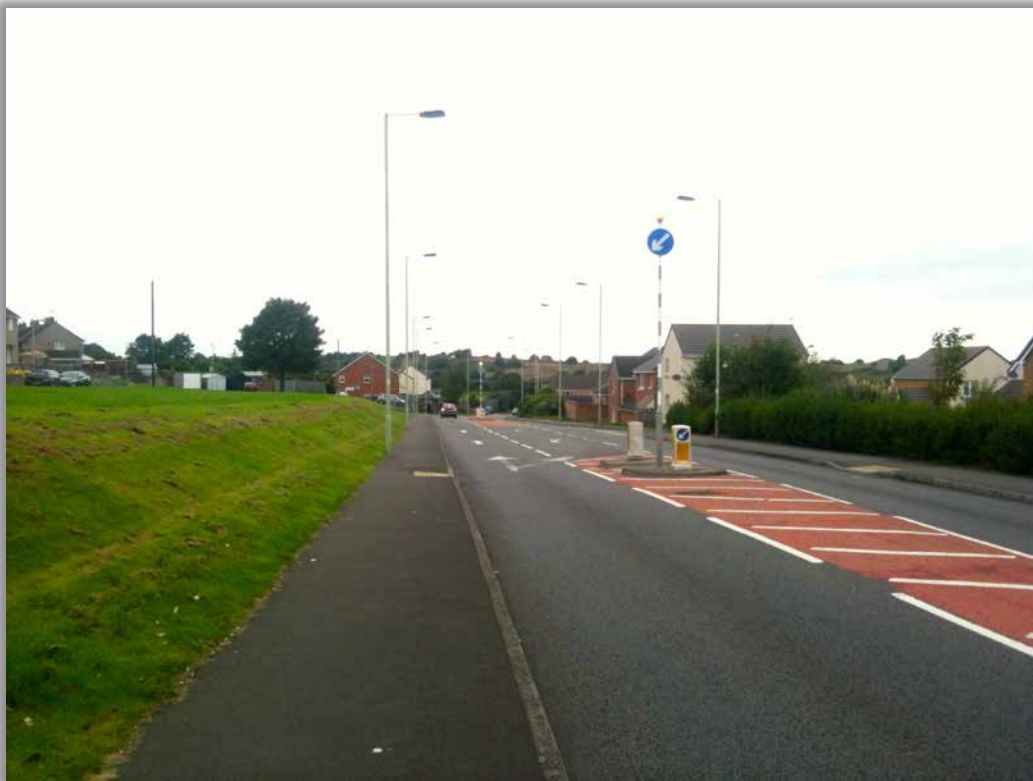
Pedestrian Refuge Beacon & Lighting Column at B4238 / Mawdlam Way Junction
