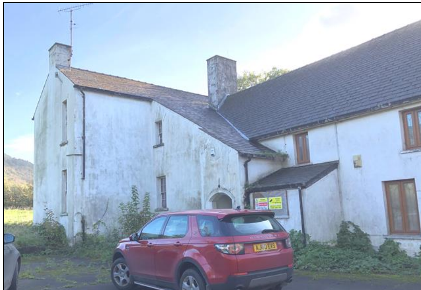
Photograph 2 – Side Elevation of Existing House
