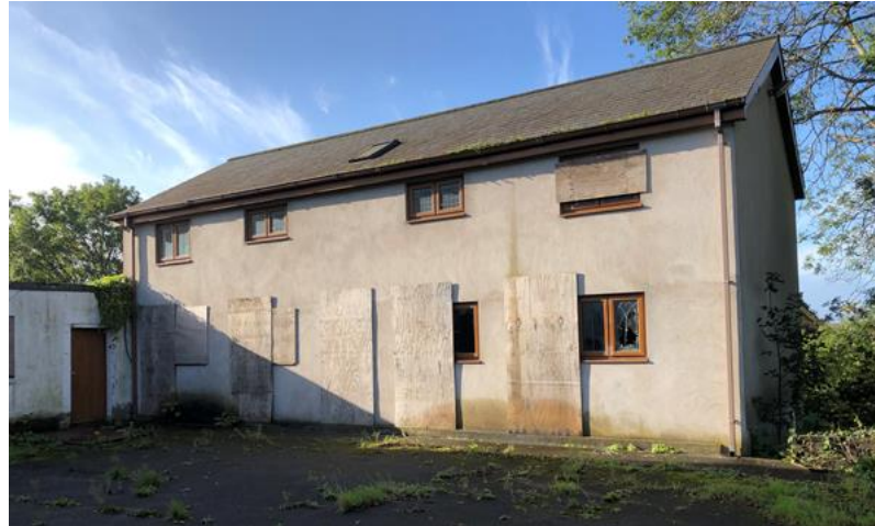
Photograph 3 – Existing Detached Two-Storey Annexe extended in 2006
