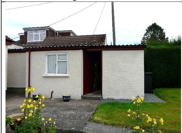
Photo 5: West facing front of garage
