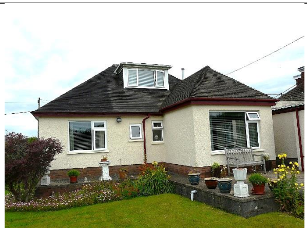
Photo 2: South facing rear
