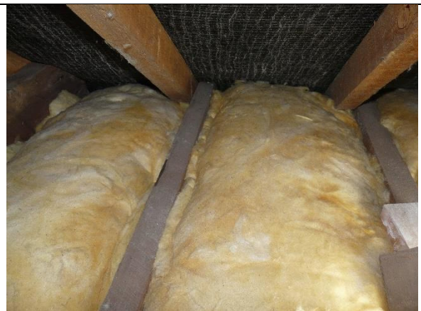
Photo 20: The loft floor is insulated with yellow fibreglass material at floor level
