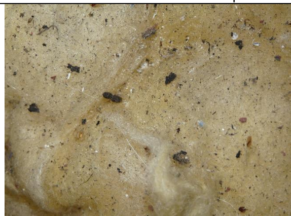
Photo 26: Close up view of bat droppings
