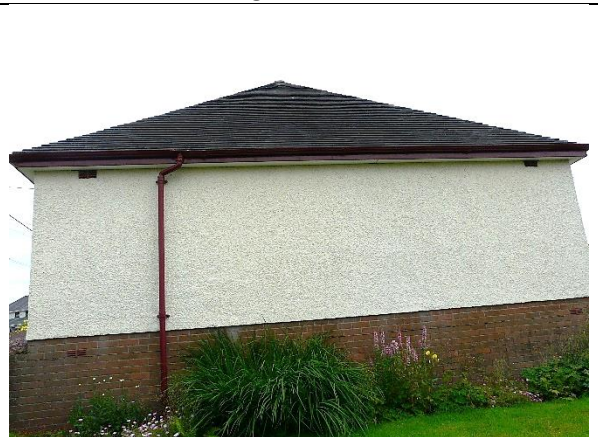
Photo 4: West facing side
