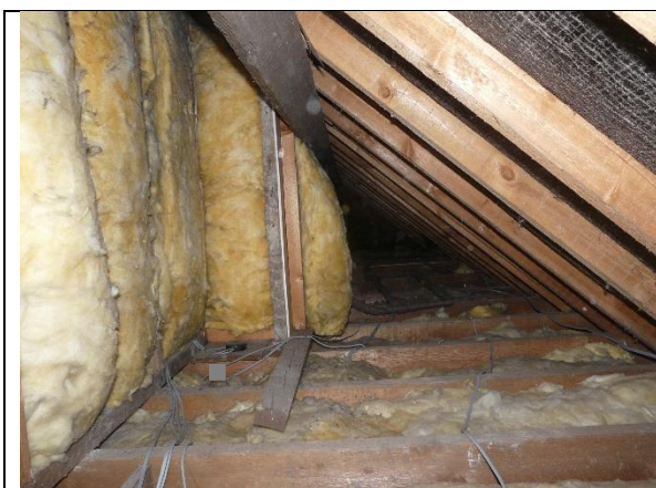
Photo 25: Internal view of eaves loft spaces
