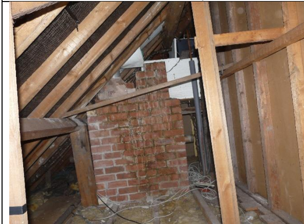
Photo 23: Internal view of loft spaces
