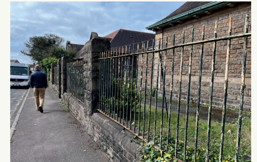
Stone walls and railings to boundary
