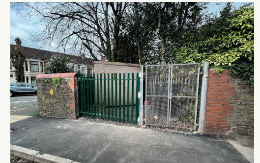
Substation and access
