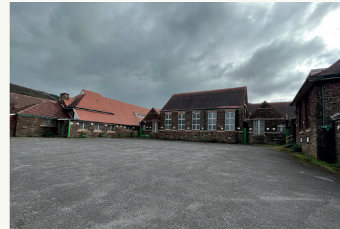
Existing school buildings - Exterior
