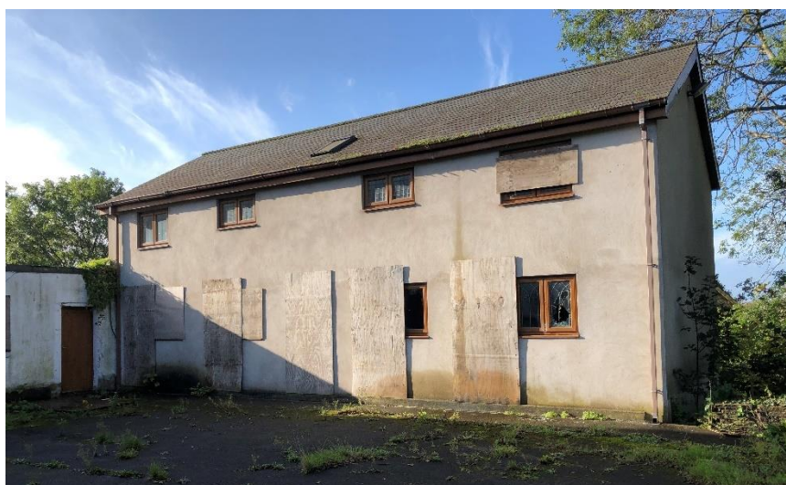
Photo 3 – view of existing detached, two-storey Annexe
