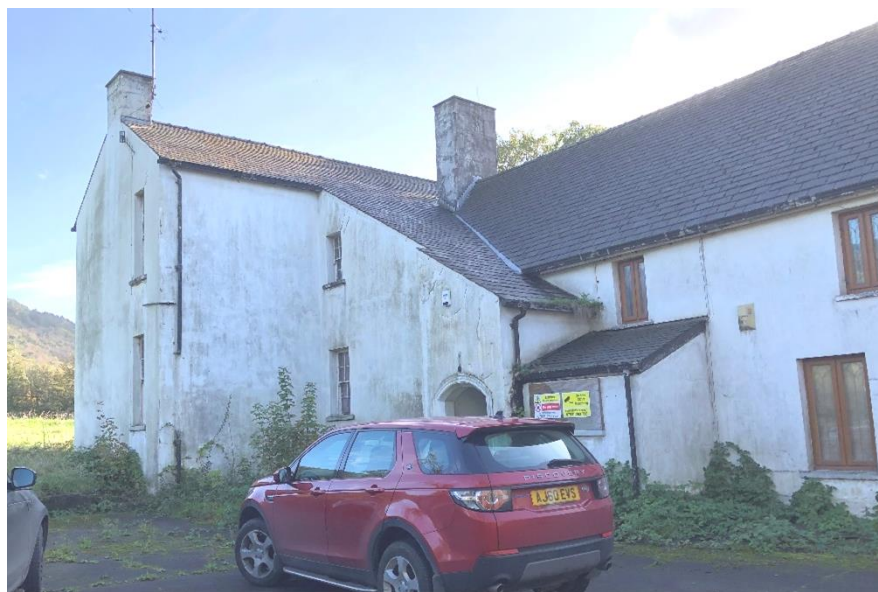
Photo 2 – view of side elevation of existing house
