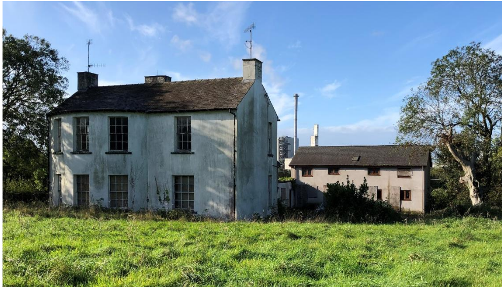
Photo 1 – view of the existing buildings at Tyn-y-Caeau
