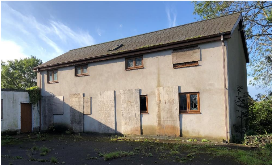
Photo 3 – view of existing detached, two-storey Annexe
