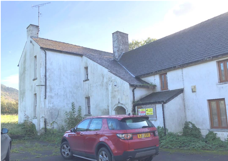
Photo 2 – view of side elevation of existing house
