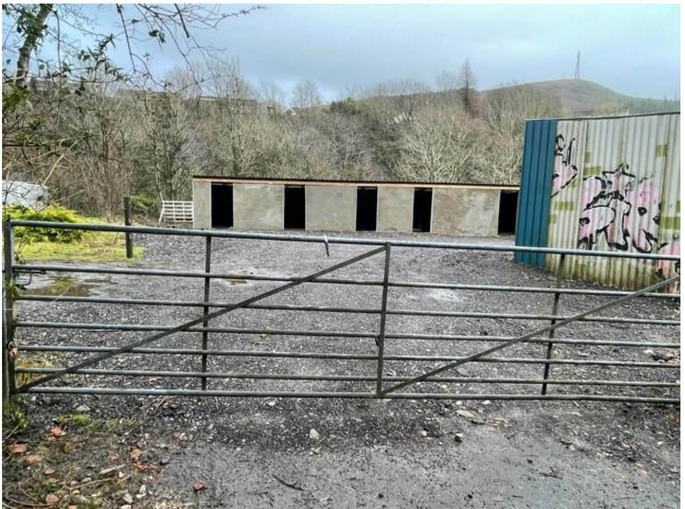
Recent photograph of the application site
