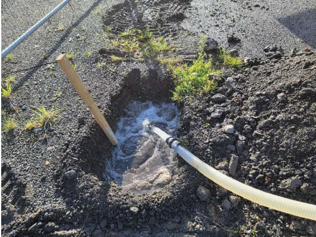
Picture 8 – Test Pit 2 test.
