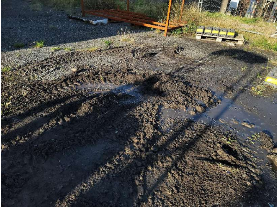
Picture 10 – Test Pit 2 reinstatement
