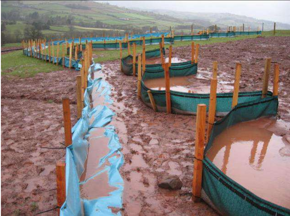
Example of Silt Fencing
