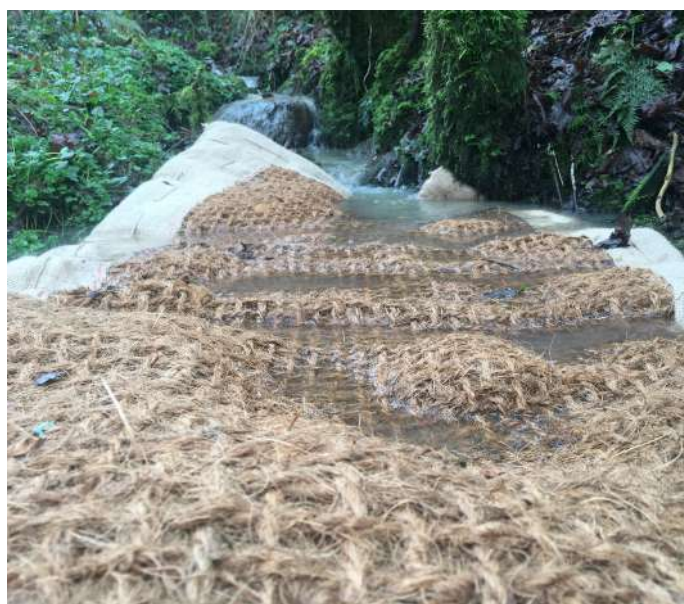
Each SiltMat can capture 40kg of sediment
