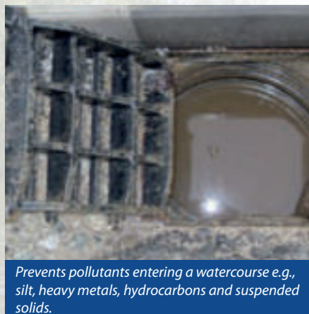
Gully Guard™ traps debris for easy collection and removal.
