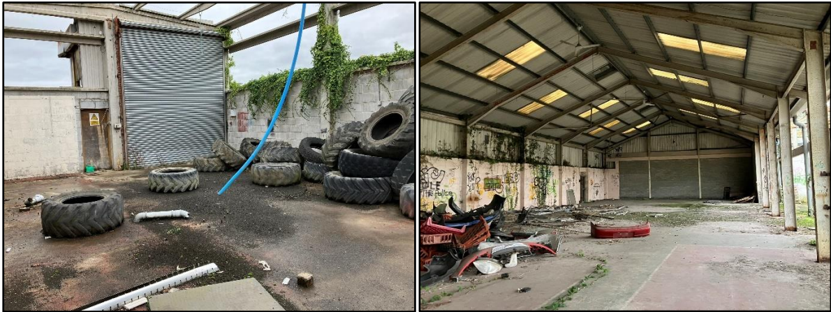
Plate 1 – Eastern Building (northern extent – left & southern extent – right)
