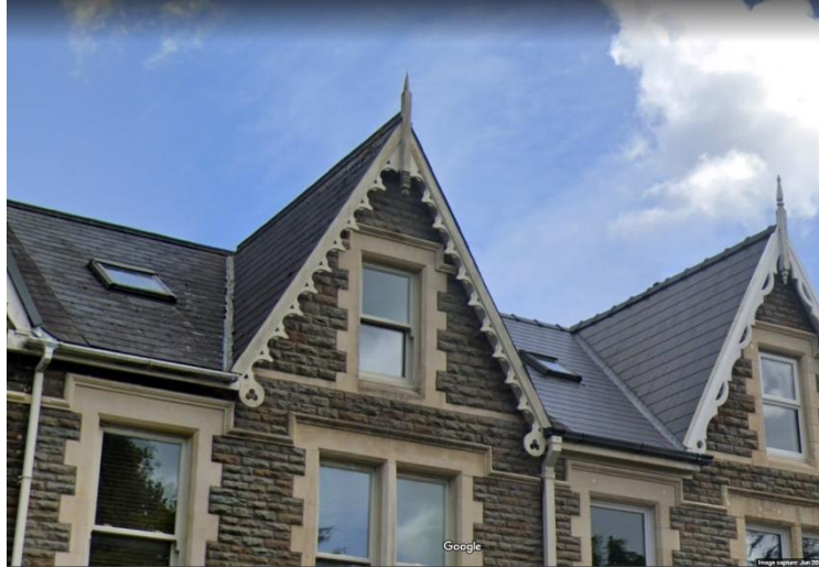
Photo 1 – Rooflights (Image courtesy of Google Streetview)
