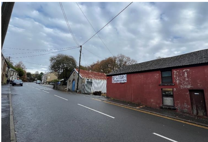
Fig. 12 – Brynaman Builders Supplies premises
