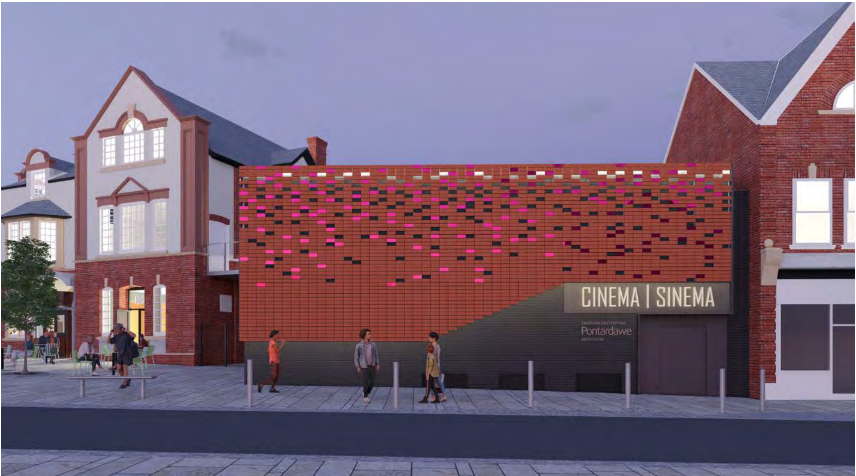
View of South-West Elevation from High Street
