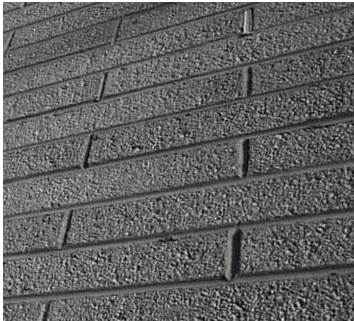
Forticrete linear blockwork for the facade base
