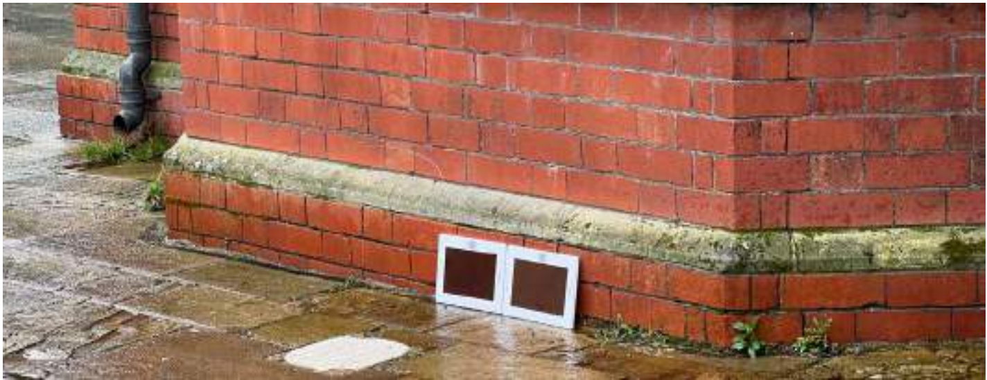
Comparison of steel finishes against external brick in wet conditions.
