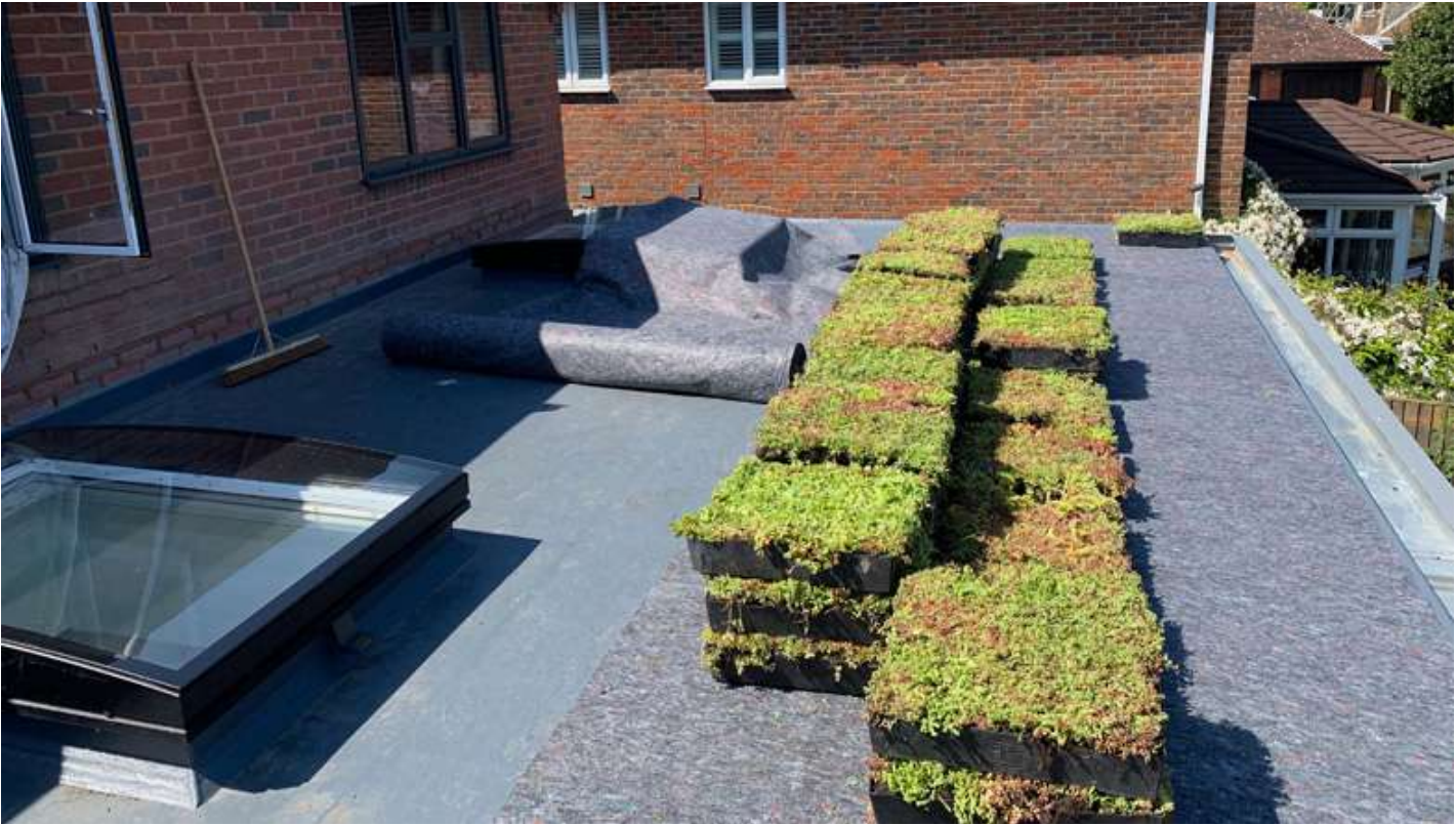
Separation and geotextile layers installed before sedum modules.
