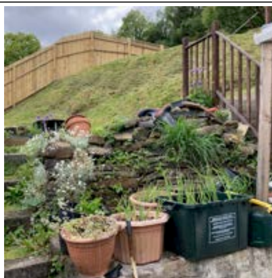
Figure 9. Dry stone wall.
