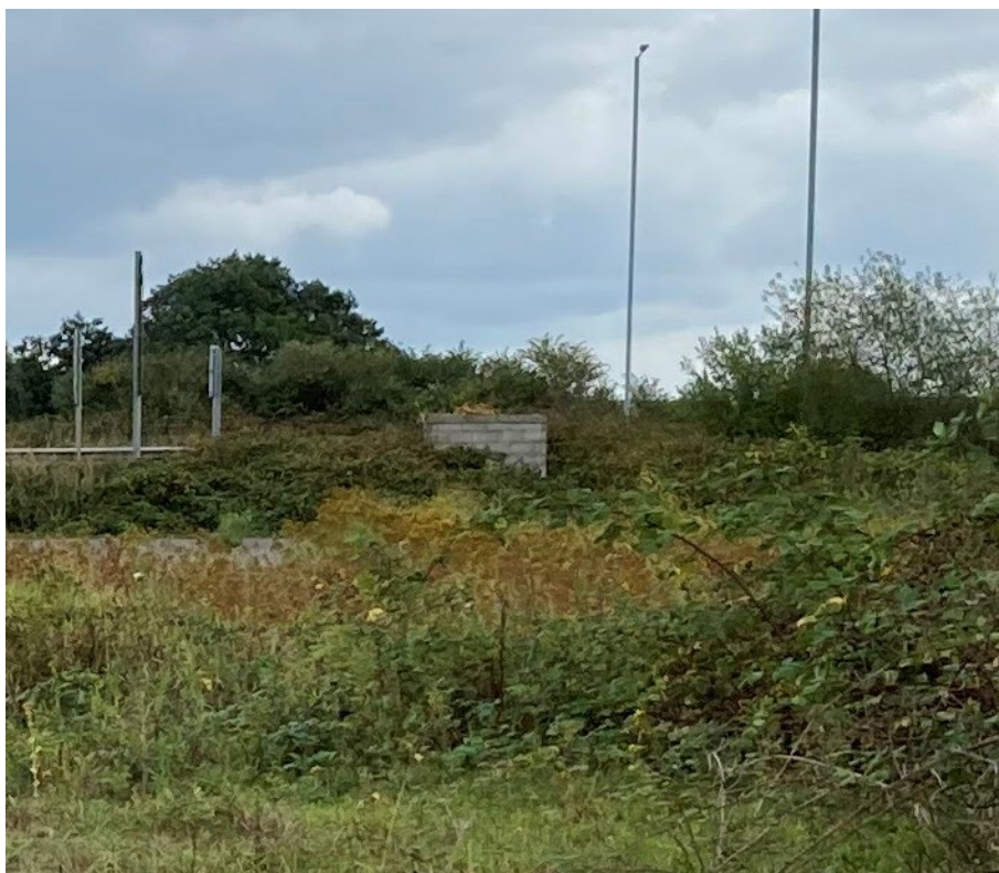
Photograph 8 - Building with negligible BRP
