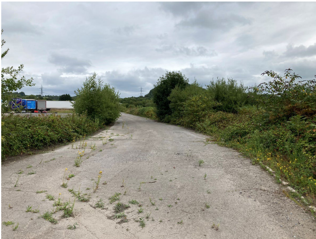
Photograph 7 - Area of hardstanding
