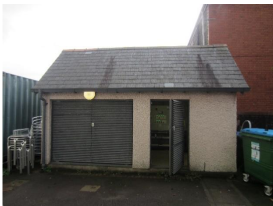
Plate 3: Gaps along edge tiles on south-west end of plant room
