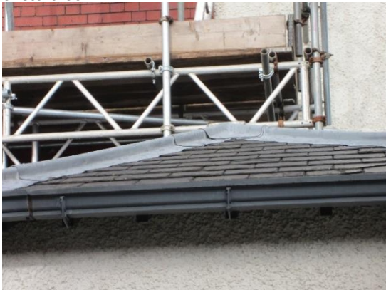
Plate 7: Lifted roof tiles and gap beneath lead flashing of storeroom
