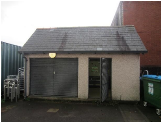
Plate 3: Gaps along edge tiles on south-west end of plant room
