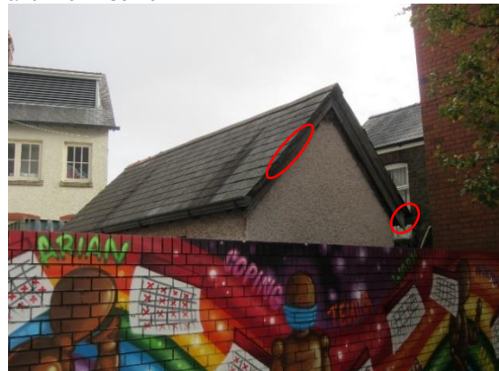
Plate 4: North-east elevation of plant room, location of bat dropping at apex and gap at edge tile
