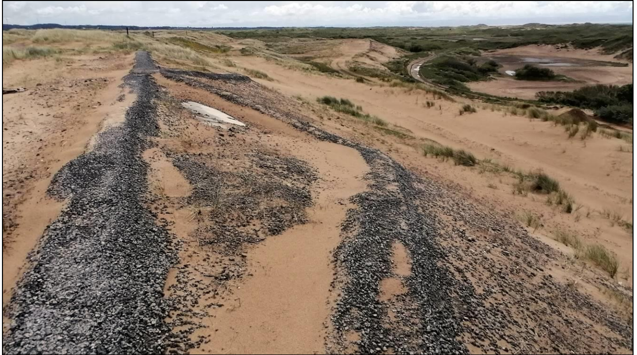
Photo 13: Area D9 landfill face exposed to prevailing winds with trial anti-erosion 16-Aug-21
