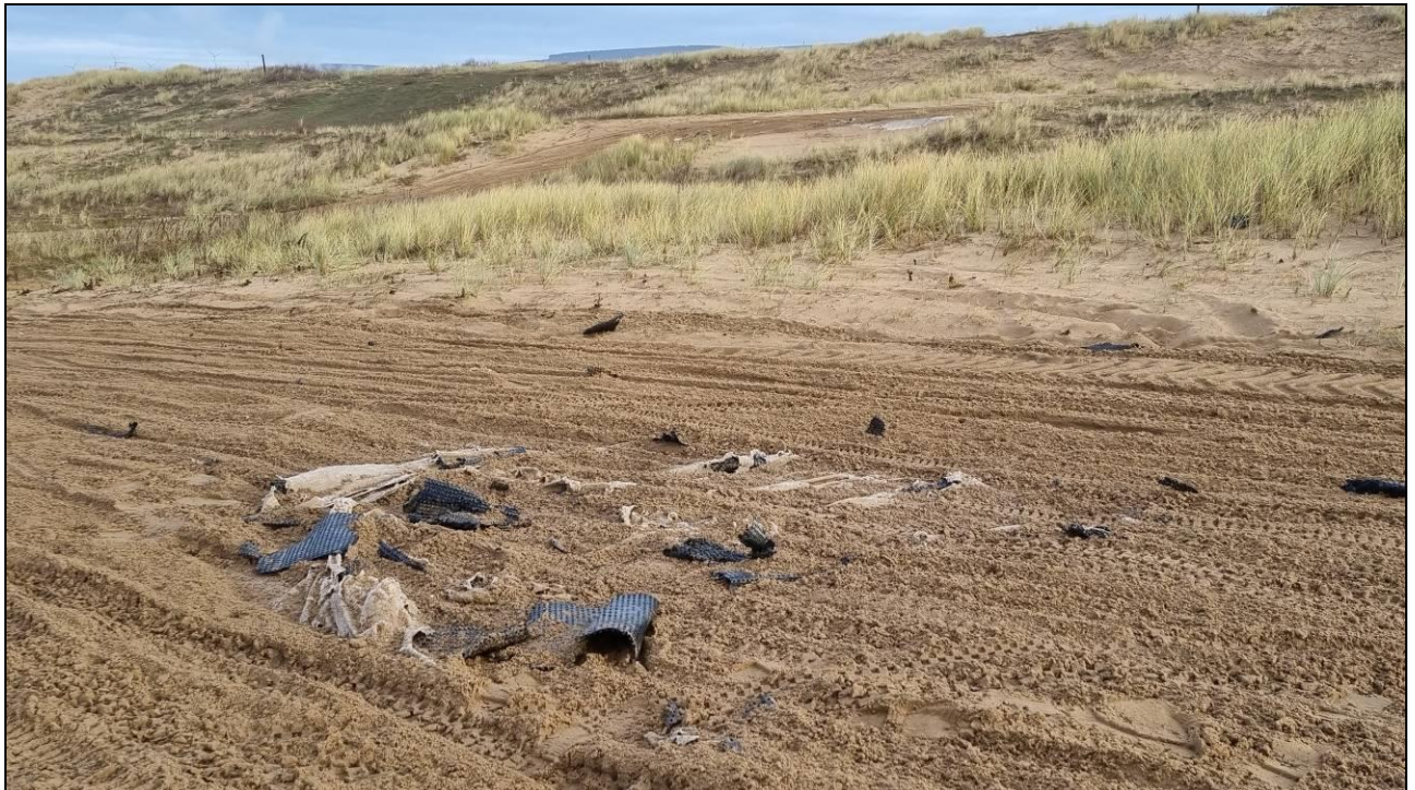
Photo 14: Area D9 part of liner damaged by off-road motor cycles 11-Jan-22
