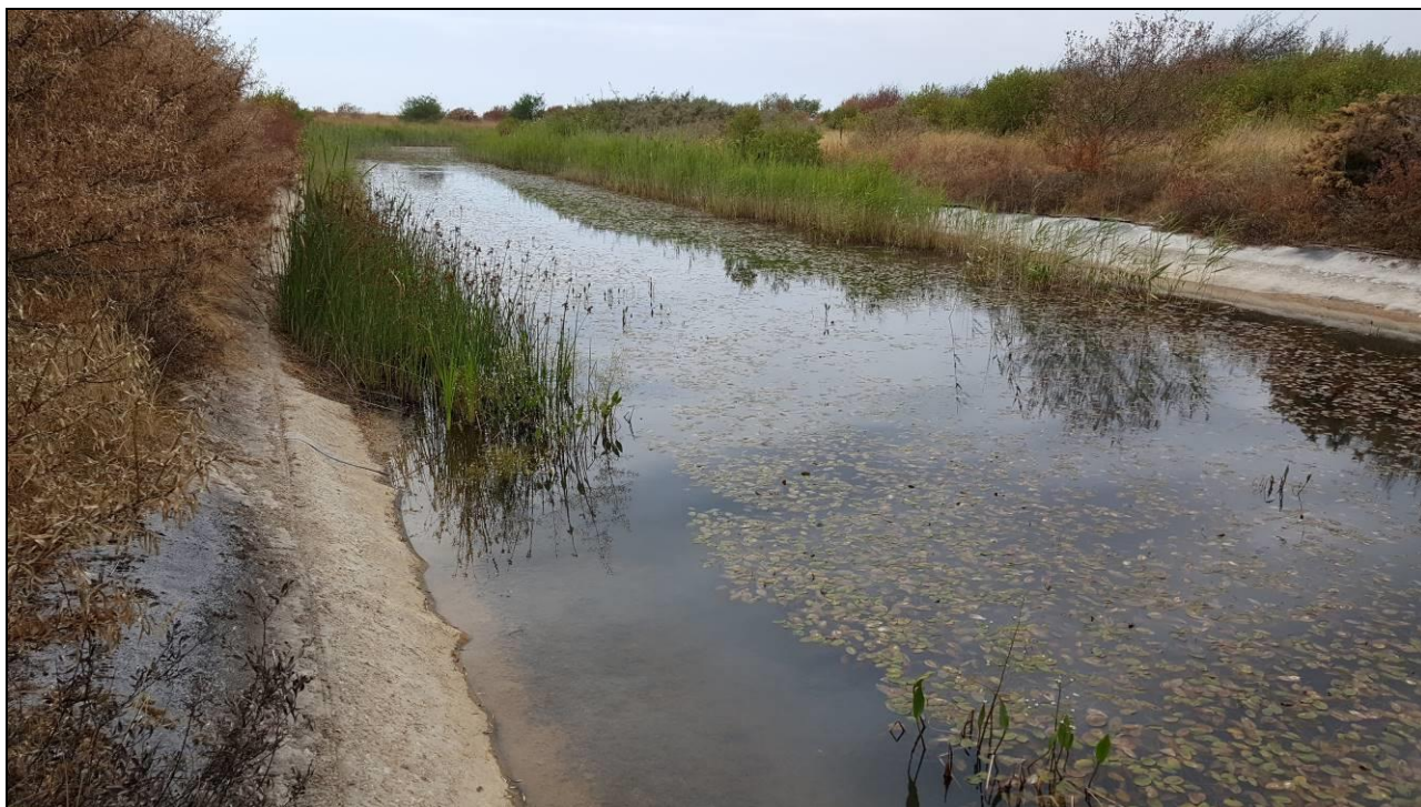
Photo 21: P4 with exposed liner, well developed emergent vegetation and scrub 26-Jul-18
