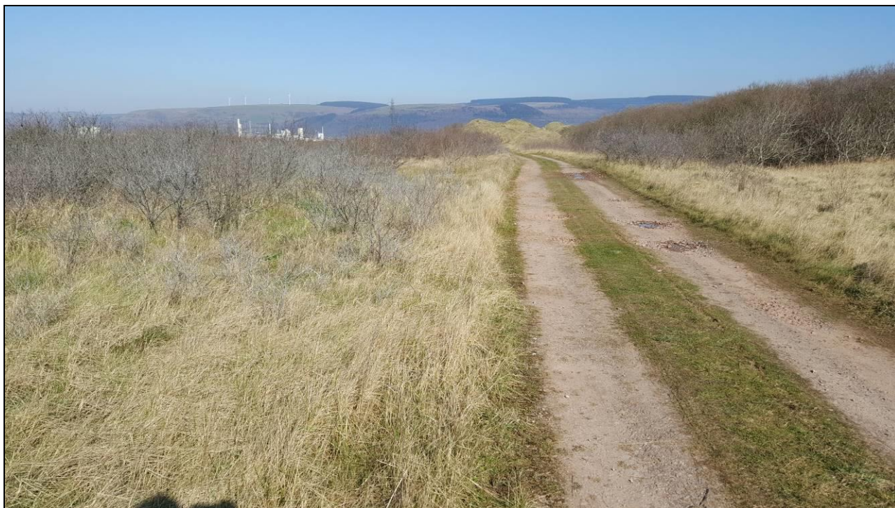
Photo 16: Area D11 scrub development on the older part of the capped landfill 26-Feb-19
