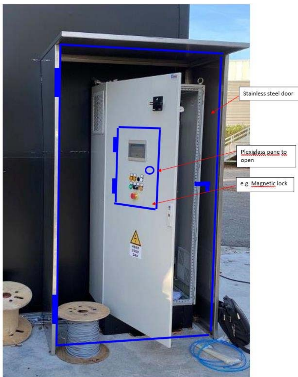
Example of the switchboard incl. housing
