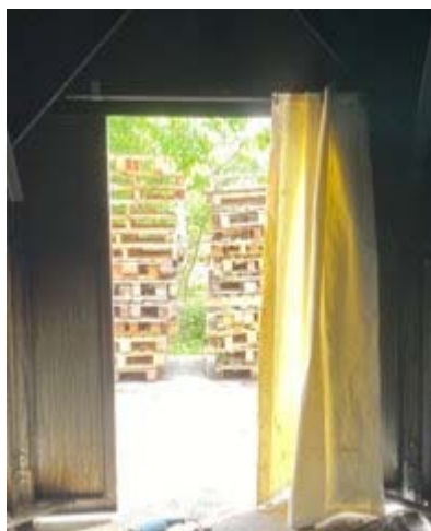
Heat resistant smoke curtains will be installed at the side entrance door and the container doors to reduce the smoke outlet to the Giraffe building during the training
