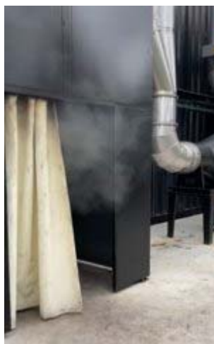
Heat resistant smoke curtains will be installed at the side entrance door and the container doors to reduce the smoke outlet to the Giraffe building during the training
