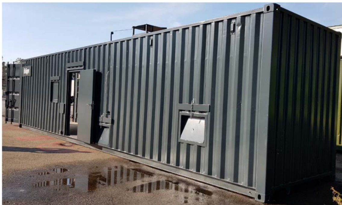
40' high cube fire training container
