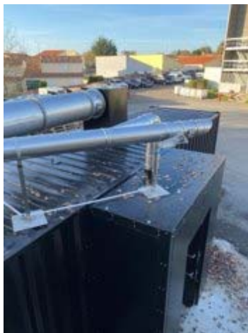
Chimney with lockable flap on the roof of the observation room covered by a special rollover extraction hood (hood made of stainless steel)
