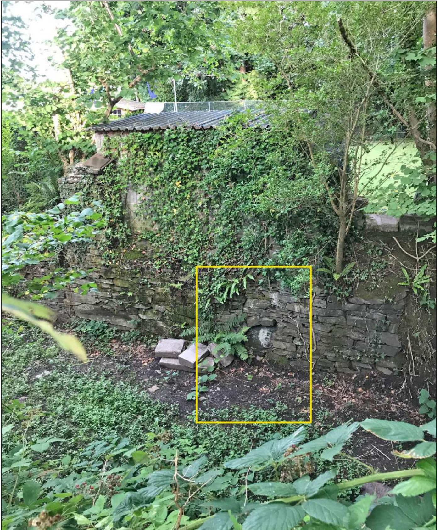
FIGURE 12 FEATURE IN FORMER RAILWAY RETAINING WALL
