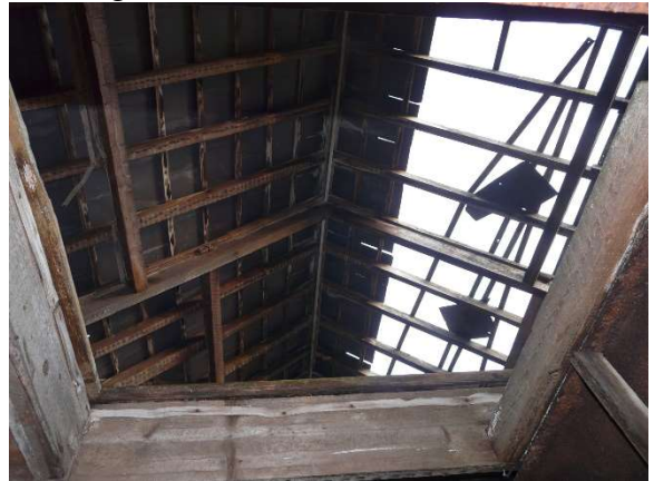
Image 11: View of roof - main section of building
