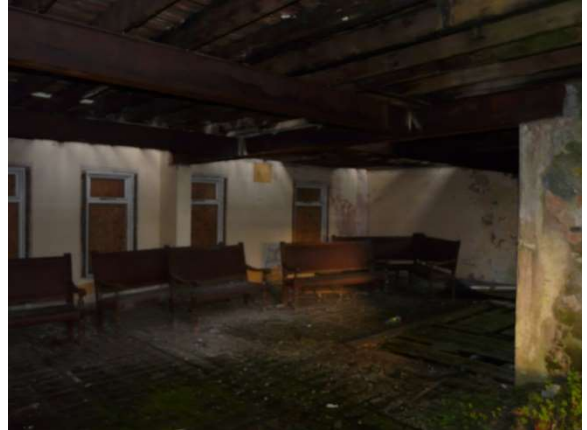
Image 10: First floor room to rear of building
