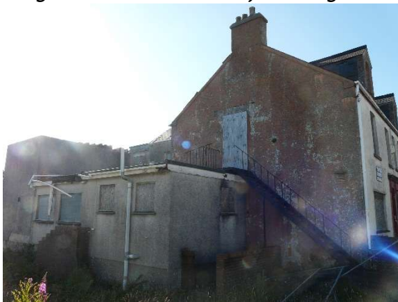
Image 3: South elevation of building
