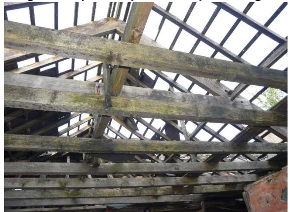
Image 12: Open roof to rear of building
