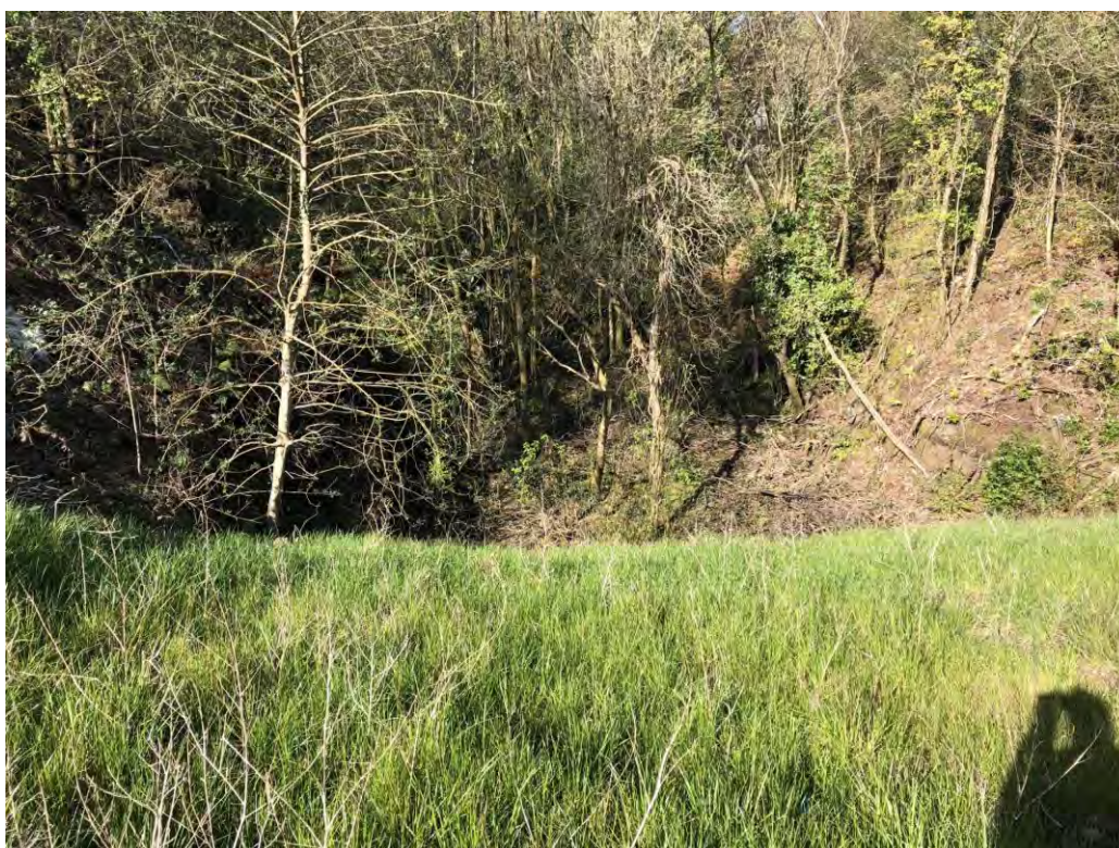
Plate 4: View of grassed fill material (foreground) within the historic railway cutting looking west.
