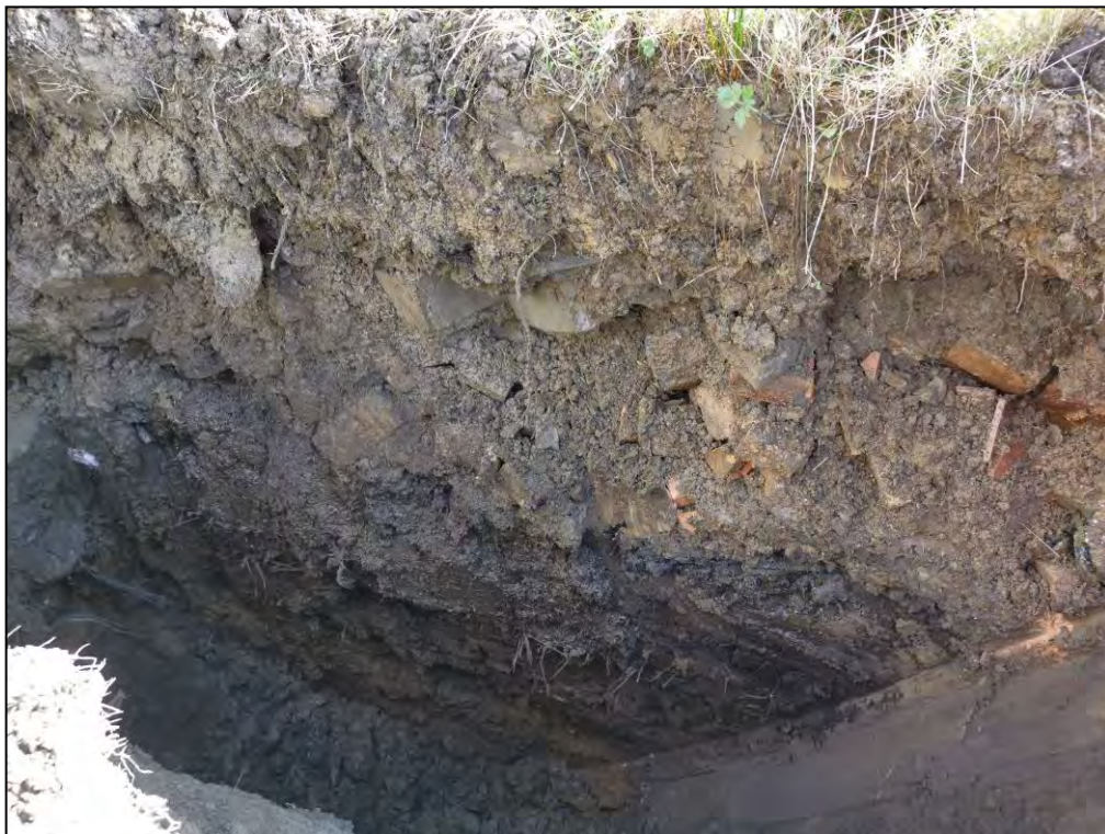
Plate 8: Fill A in upper portions of trial pit (TP08), man-made constituents including brick and concrete visible.
