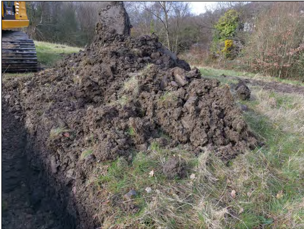
Plate 7: Fill A material arisings excavated from TP03 in the area of the former railway cutting.
