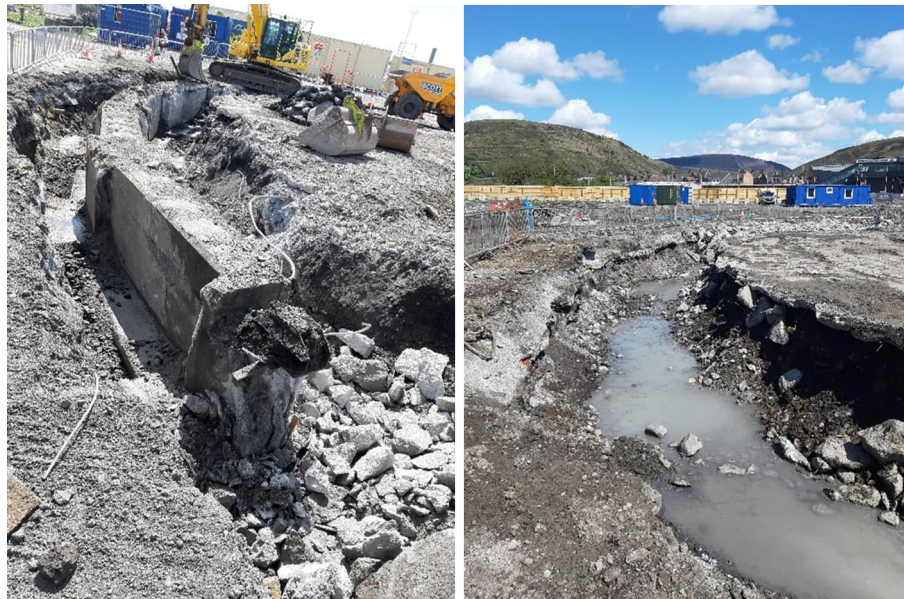
Left - Reinforced concrete ring-beam encircling gasholder. Right – Excavation following removal of ring beam.
