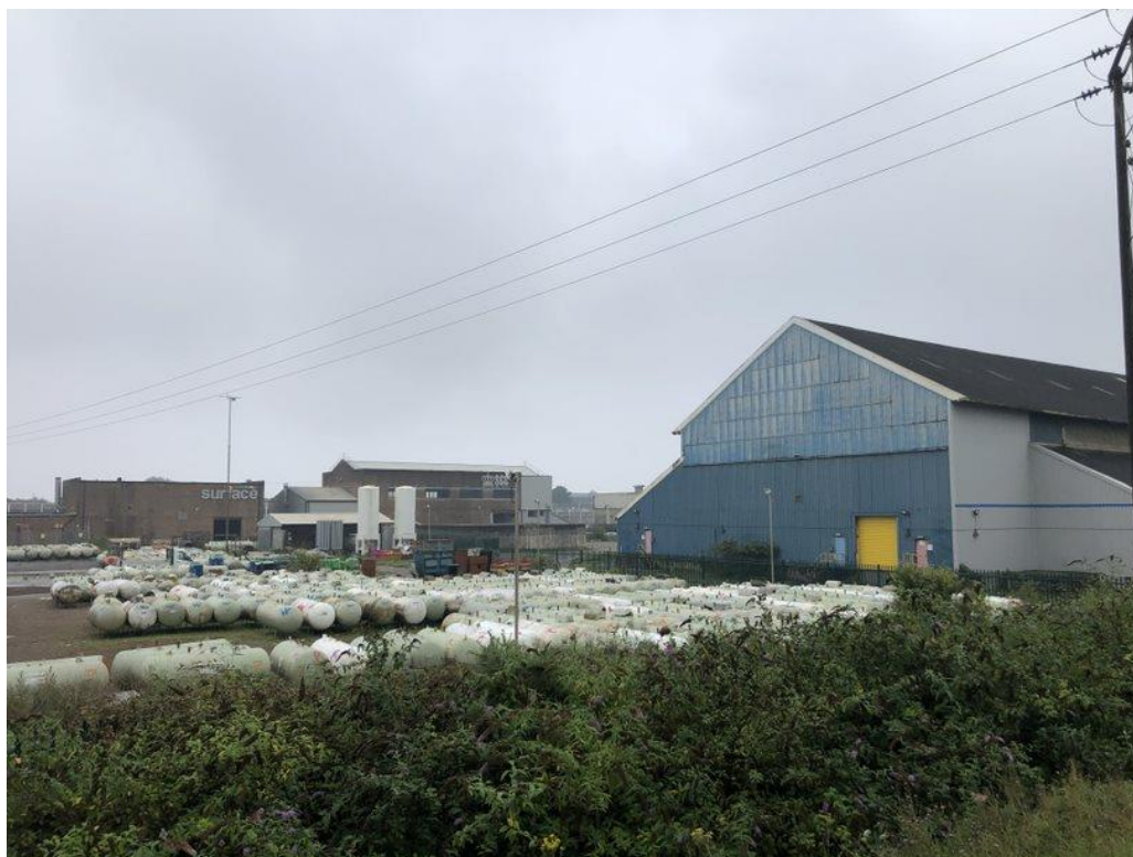
Insert 3: General View of Site Looking South West (14.08.20)
