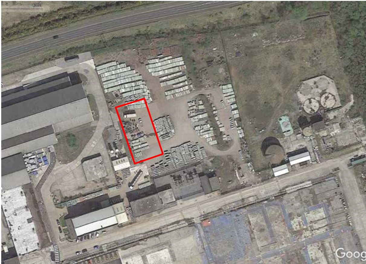
Figure 2: Aerial View showing proposed Shed footprint
