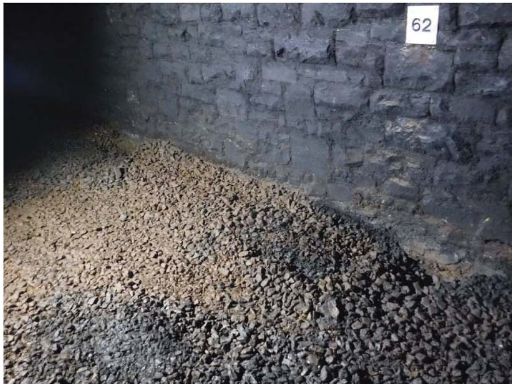
Photo No.37: 061+19 to 062+00 Solum Down, 2No. trial pits. Partially backfilled.
