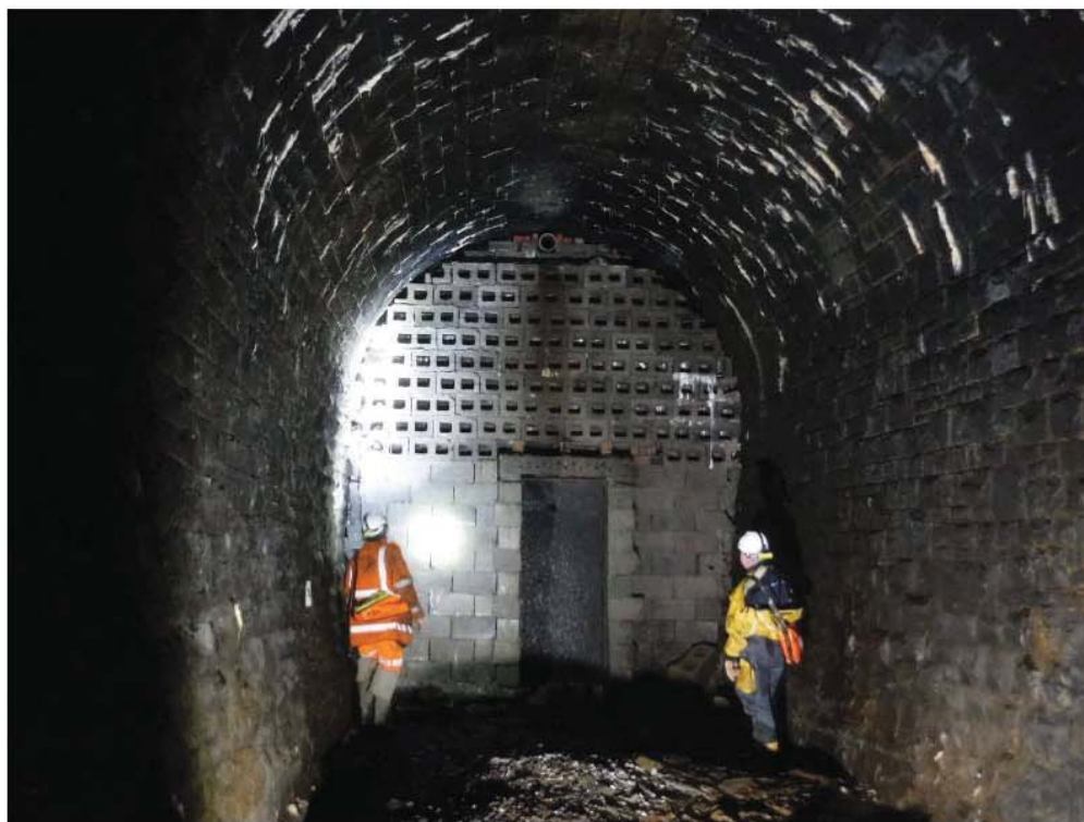
Photo No.46: 073+05 Portal Up & Down, View of blocked up Abergwynfi Portal from inside tunnel.
