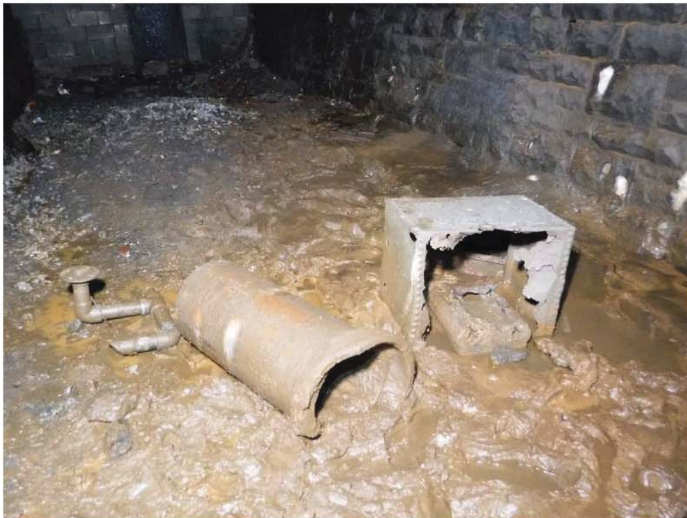
Photo No.45: 072+11 to 073+05 Solum Up & Down, Debris.
