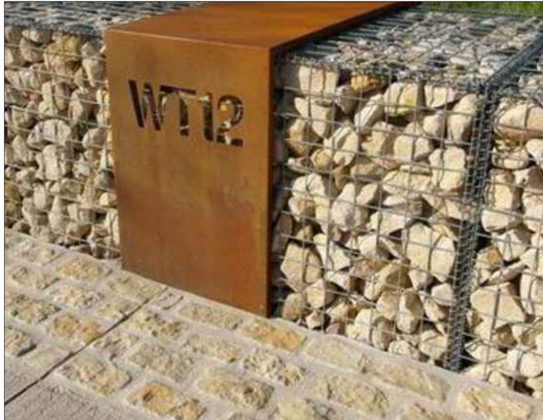
2 GABION AND WEATHERED STEEL BENCHES
