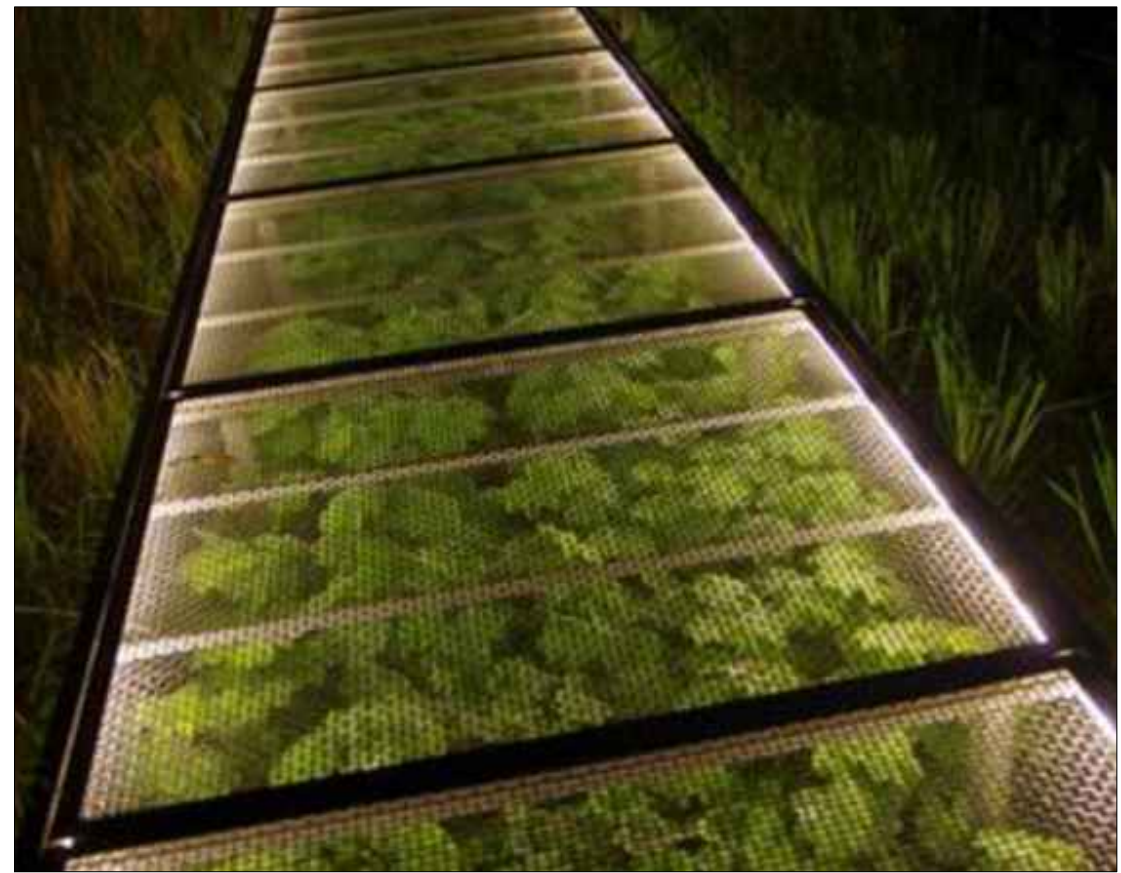
4 METAL GRATE WALKWAY WITH LIGHTING
