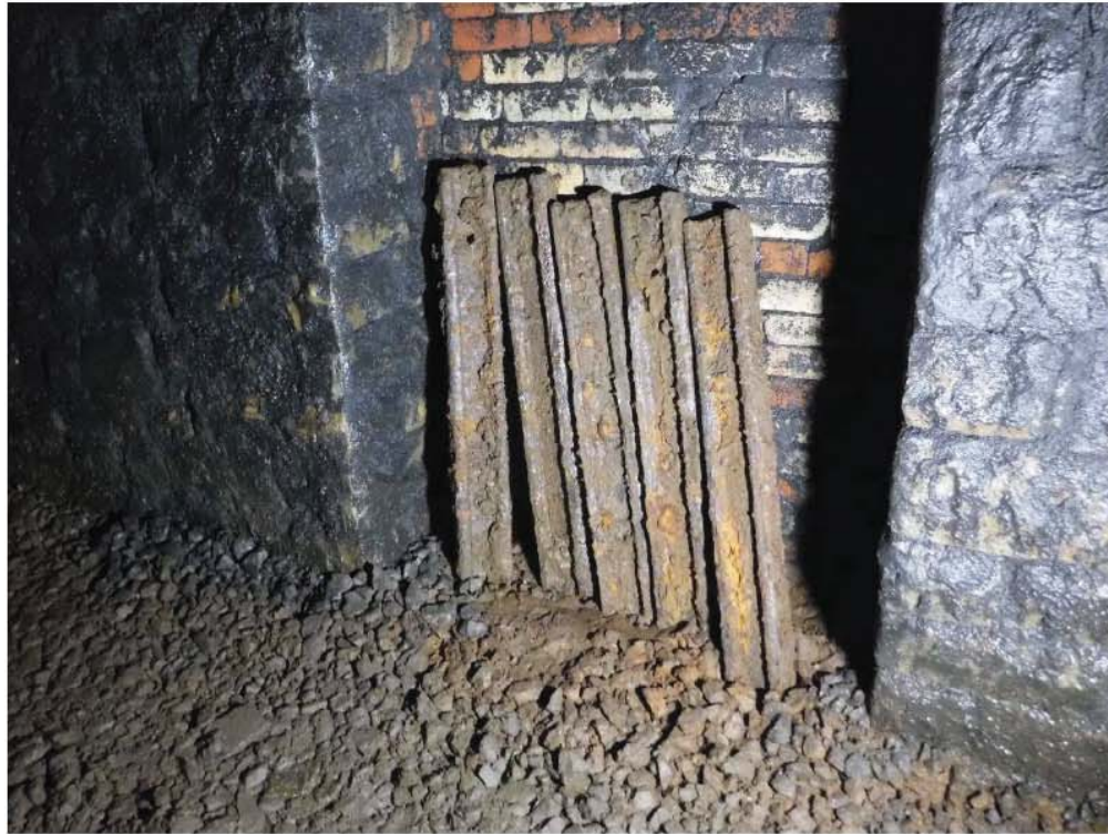
Photo No.14: Full Length of Tunnel, Solum Up & Down, drainage WIP, rail irons from broken out catch-pits & new construction materials found in refuges.
