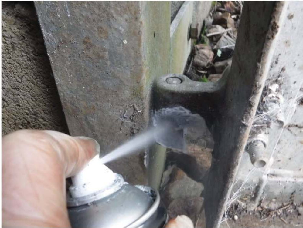
Photo No.6: Bridgend Portal, oiling door hinges.
