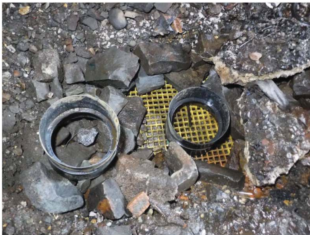
Photo No.16: Bridgend Portal, Solum Up & Down, drainage WIP, new cover found in 6'.
