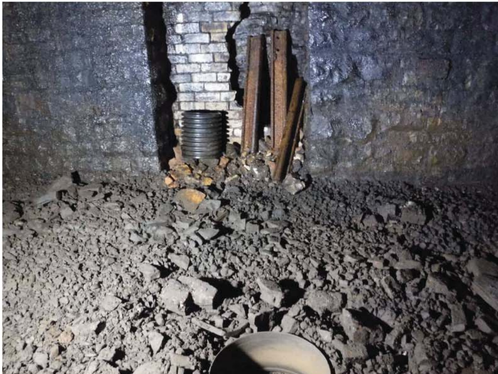
Photo No.13: Full Length of Tunnel, Solum Up & Down, drainage WIP, rail irons from broken out catch-pits & new construction materials found in refuges.
