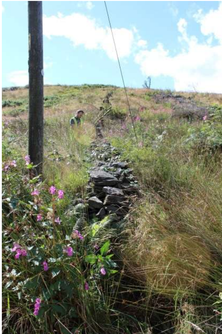
FEATURE 3: Dry stone wall. View south.
