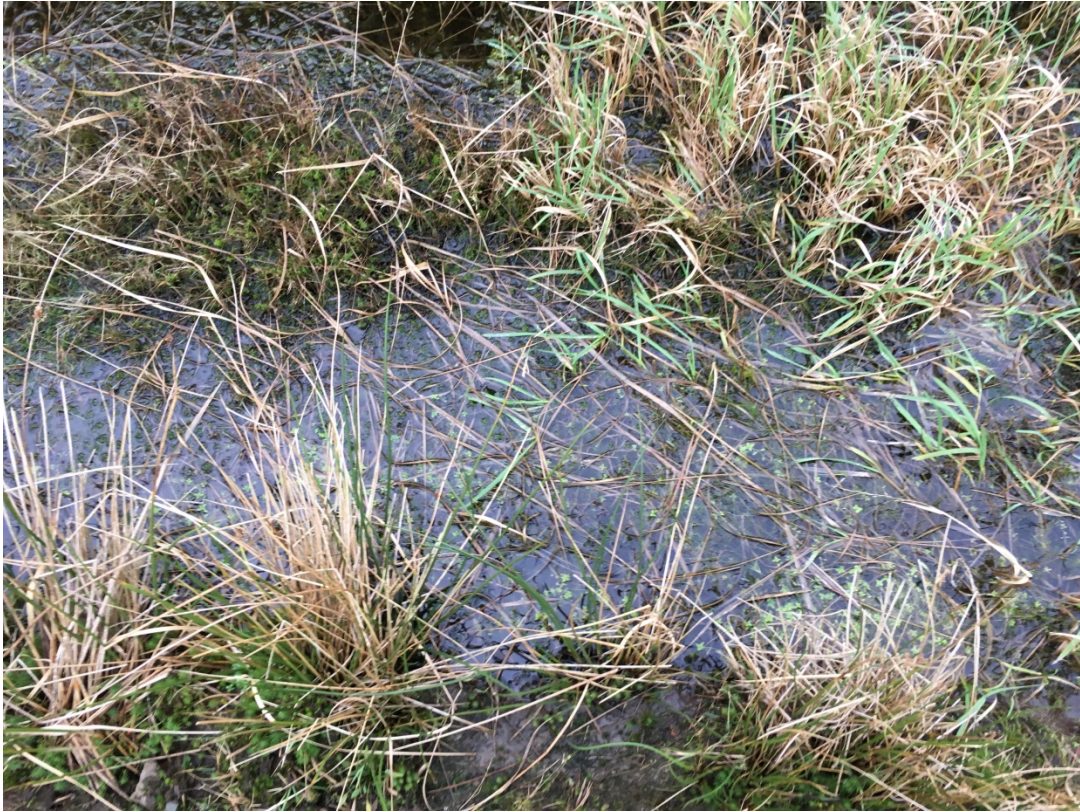
L8 Standing water along track
