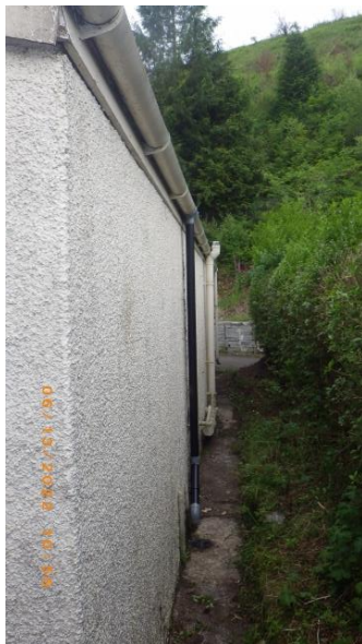
West elevation of the changing rooms
