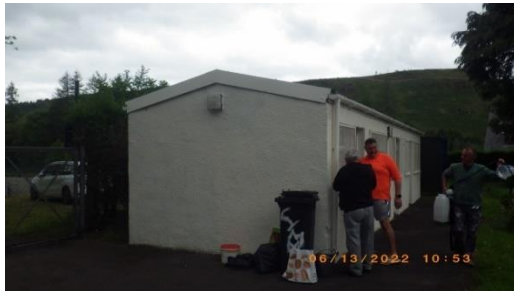
South and east elevation of the changing room
