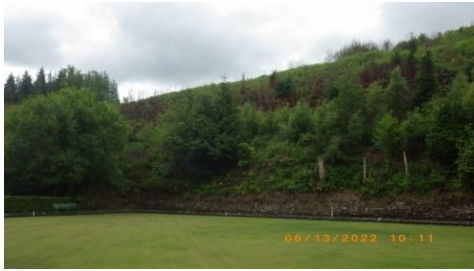
Bowling green and well vegetated slope to the south
