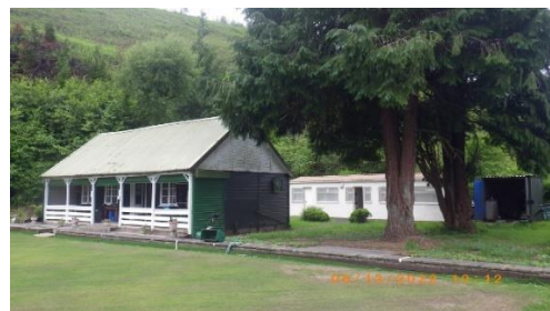
Pavilion and changing room viewed from the east
