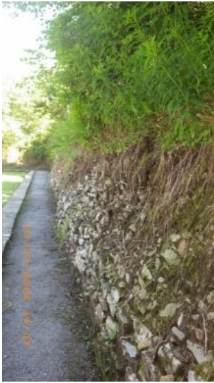
Retaining wall along the south boundary
