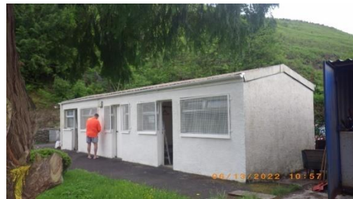
North and east elevation of the changing room
