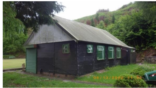
North and west elevation of the pavilion
