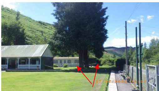
Area north of the Pavilion and changing room which is to be extended into
