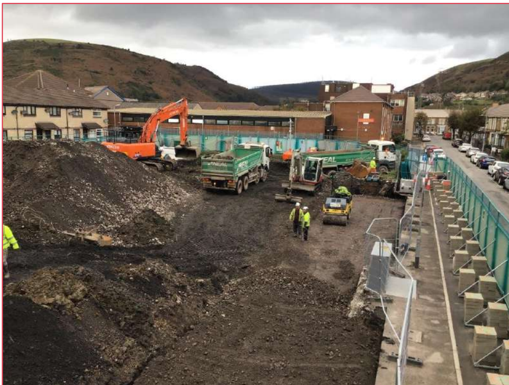
Photo 4: Reduced dig ongoing, offsite disposal (Neals) and laying of imported stone
