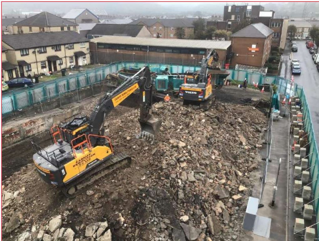
Photo 1: Demolition of northern end of existing Plaza building
