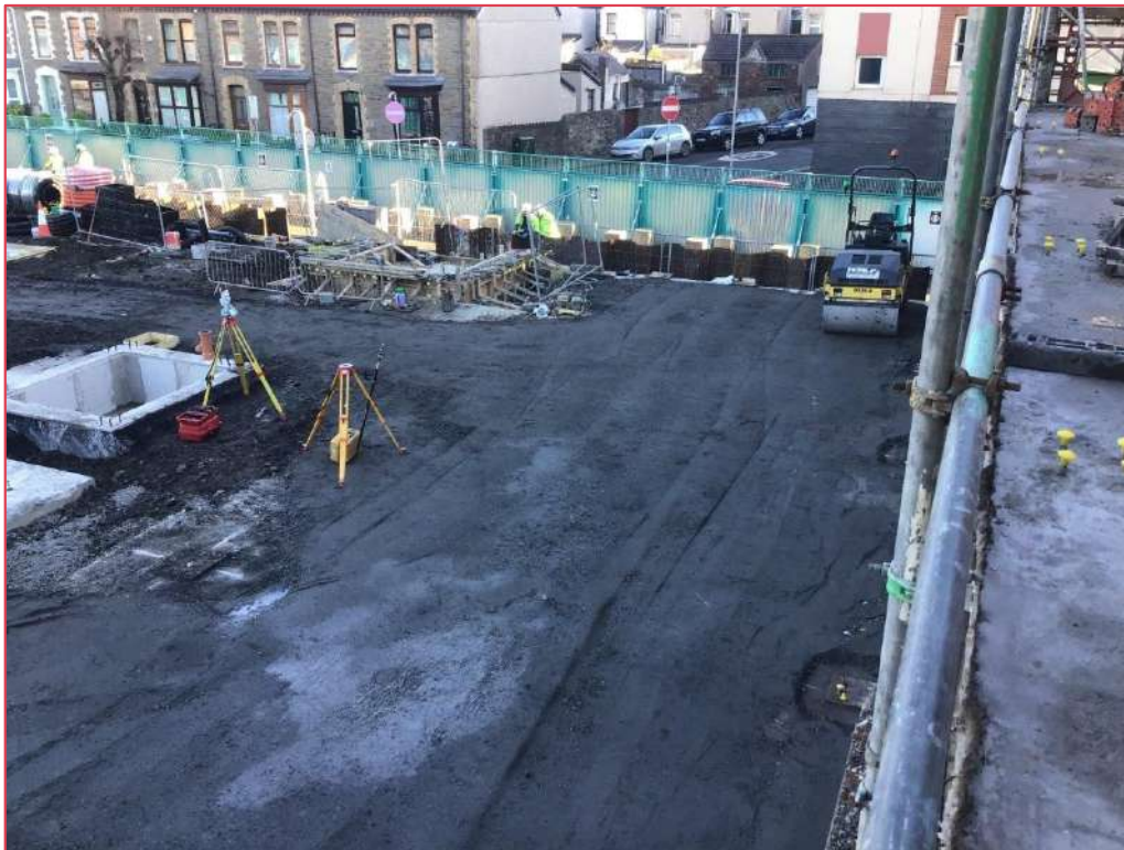
Photo 5: Levels being brought up using imported engineered stone
