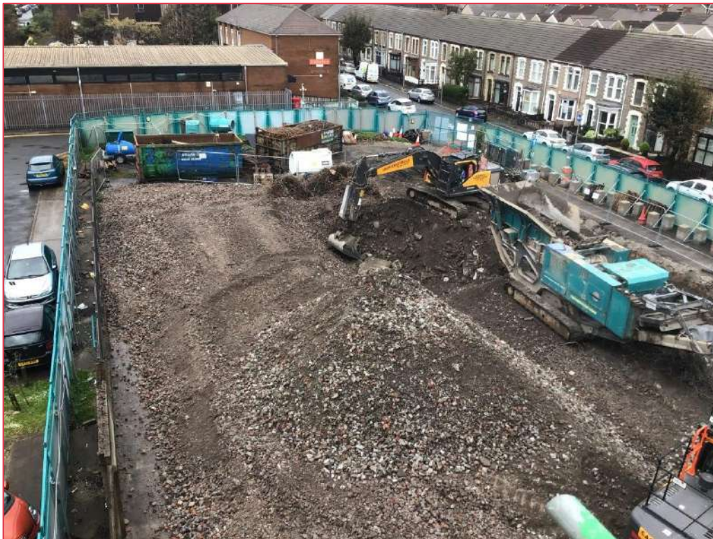
Photo 3: Reduced dig ongoing and removal offsite
