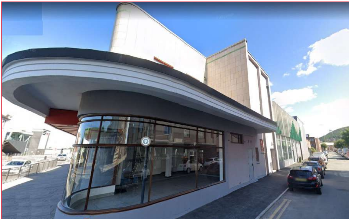
Photo 2: Completed Development - East Elevation (Eagle Street)
