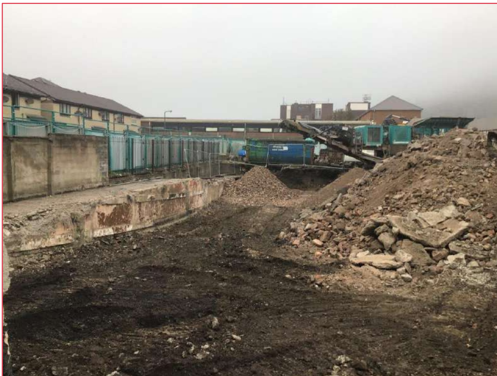
Photo 2: Reduced dig of existing soils & demolition stockpile for screening, crushing and offsite disposal
