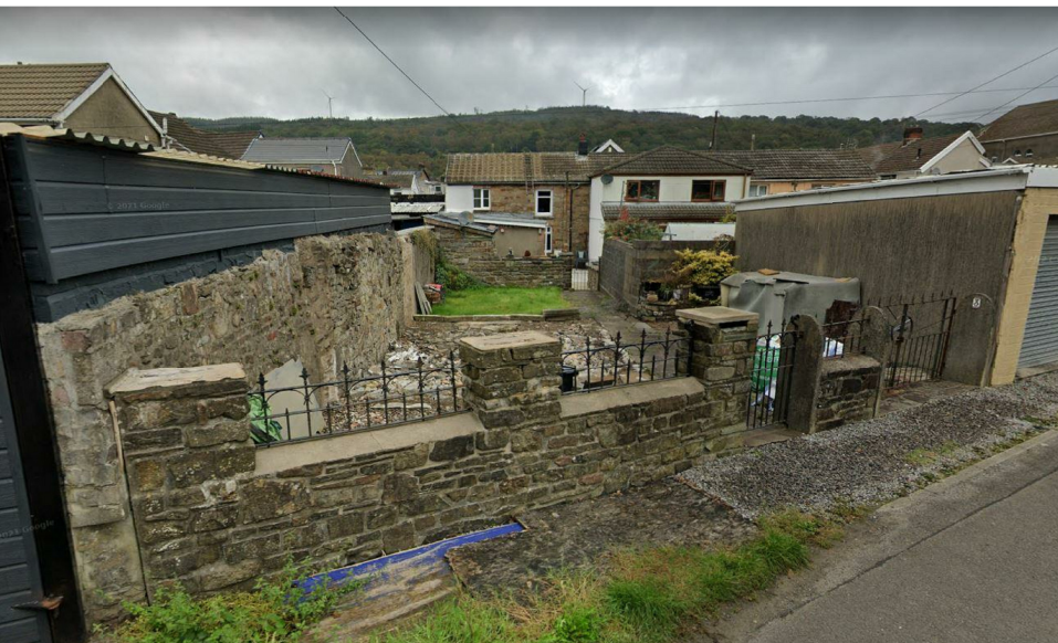
Existing Front Elevation Image 1
