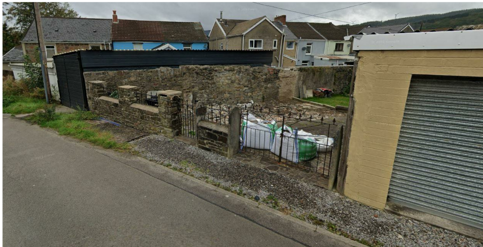
Existing Front Elevation Image 2
