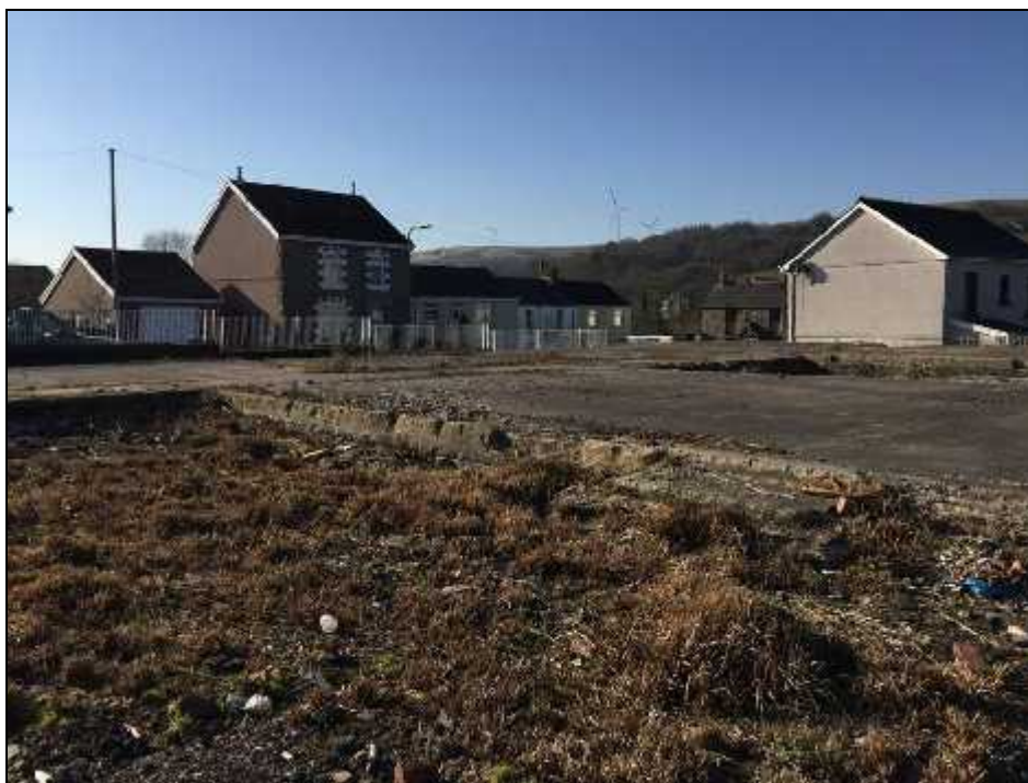
Figure 8. Concrete base of former school buildings, with strimmed vegetation in foreground
