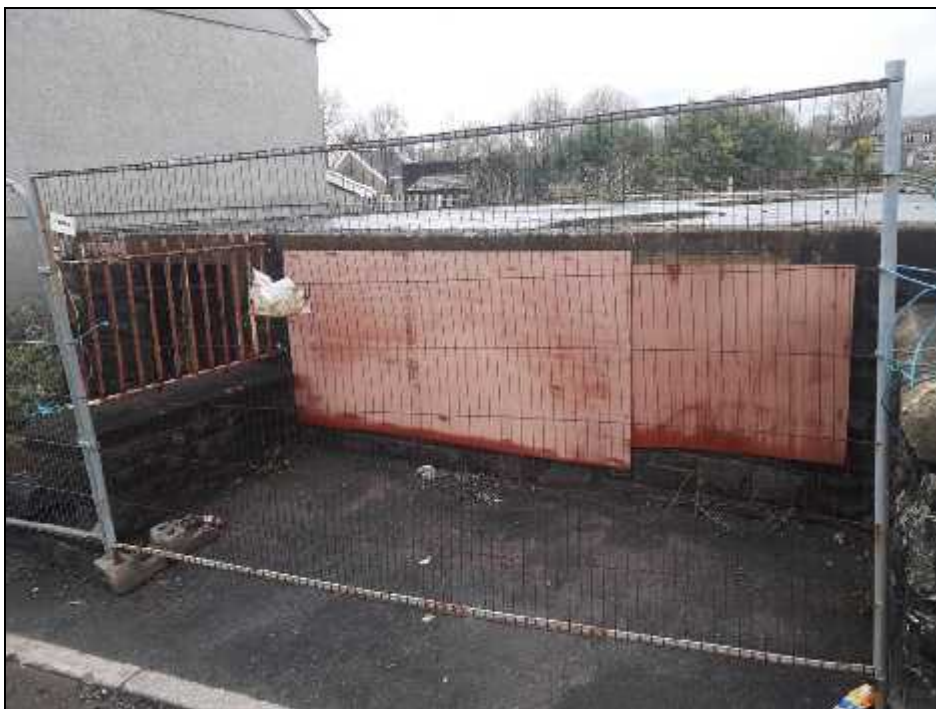
Figure 10. Former basement building
