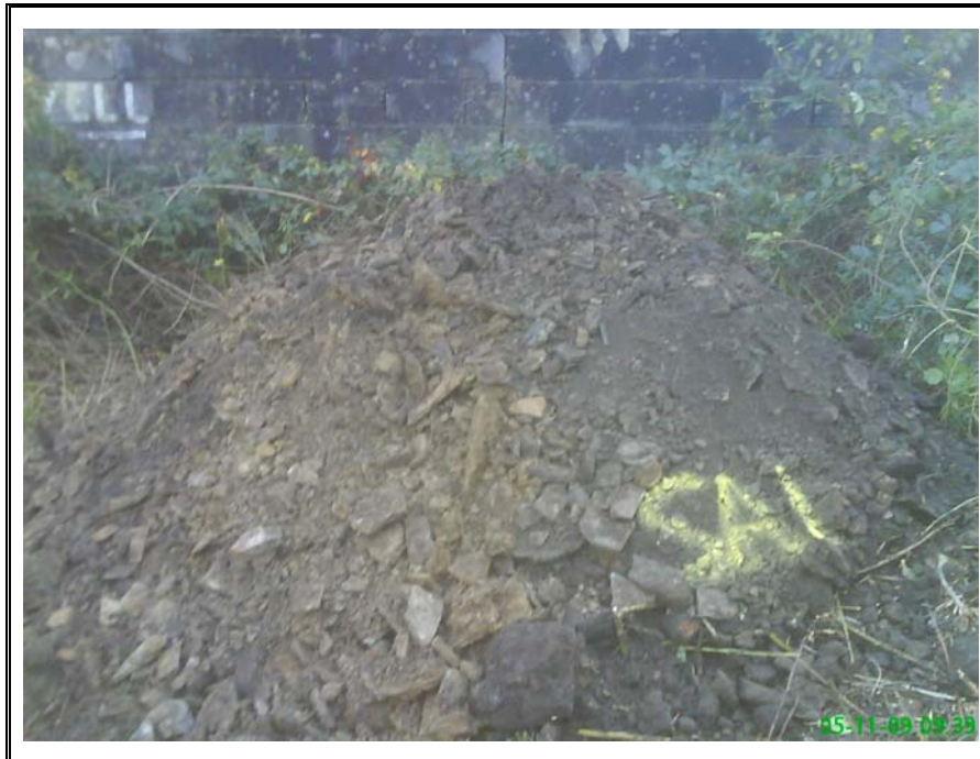
Trial Pit SA1 – Arisings
