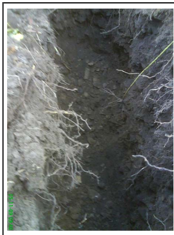
Trial Pit SA1 – Excavation.
