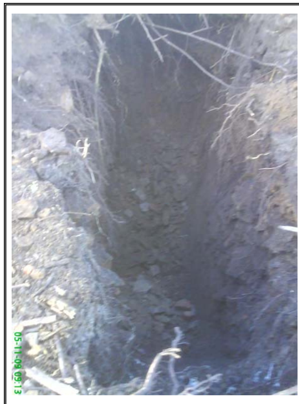
Trial Pit SA3a - Excavation
