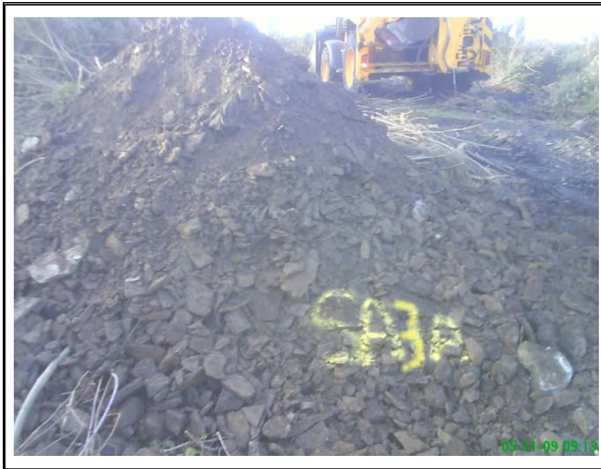
Trial Pit SA3a - Arisings.
