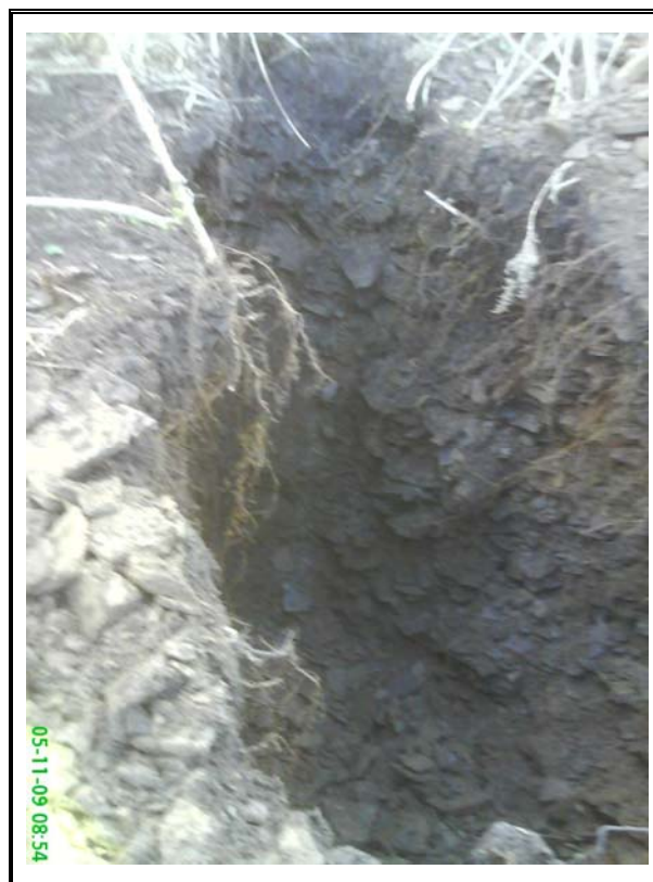
Trial Pit SA2 – Excavation.
