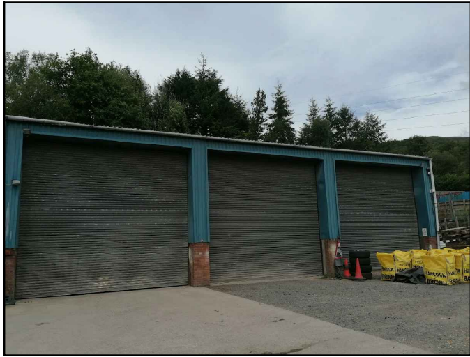
Photograph 3 Showing existing building
