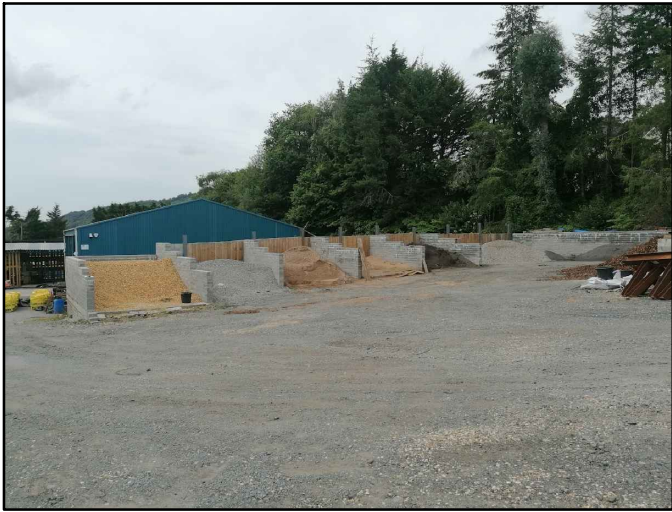
Photograph 1 Showing loading bays
