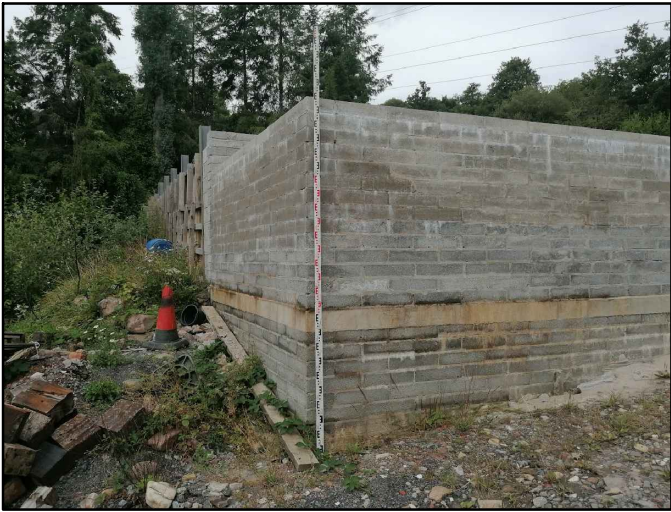
Photograph 2 Showing loading bays
