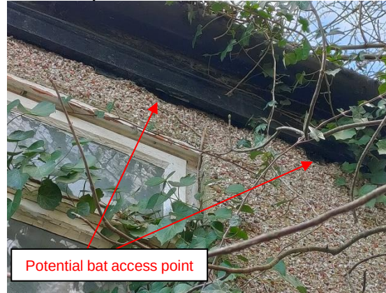
Plate 12: Gaps at barge boards on western gable 2
