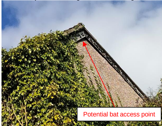
Plate 11: Gaps at barge boards on western gable 1
