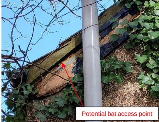
Plate 13: Gaps behind fascia boards on south elevation
