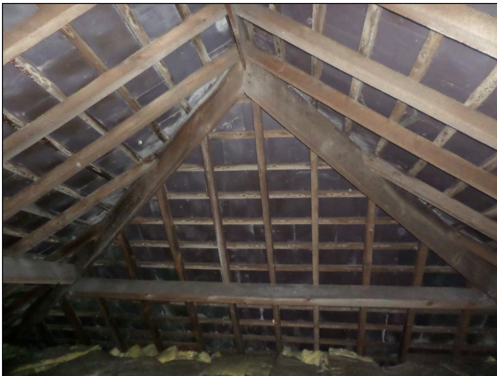
Photo 9: Exposed wooden rafters, purlins and roof slates.
