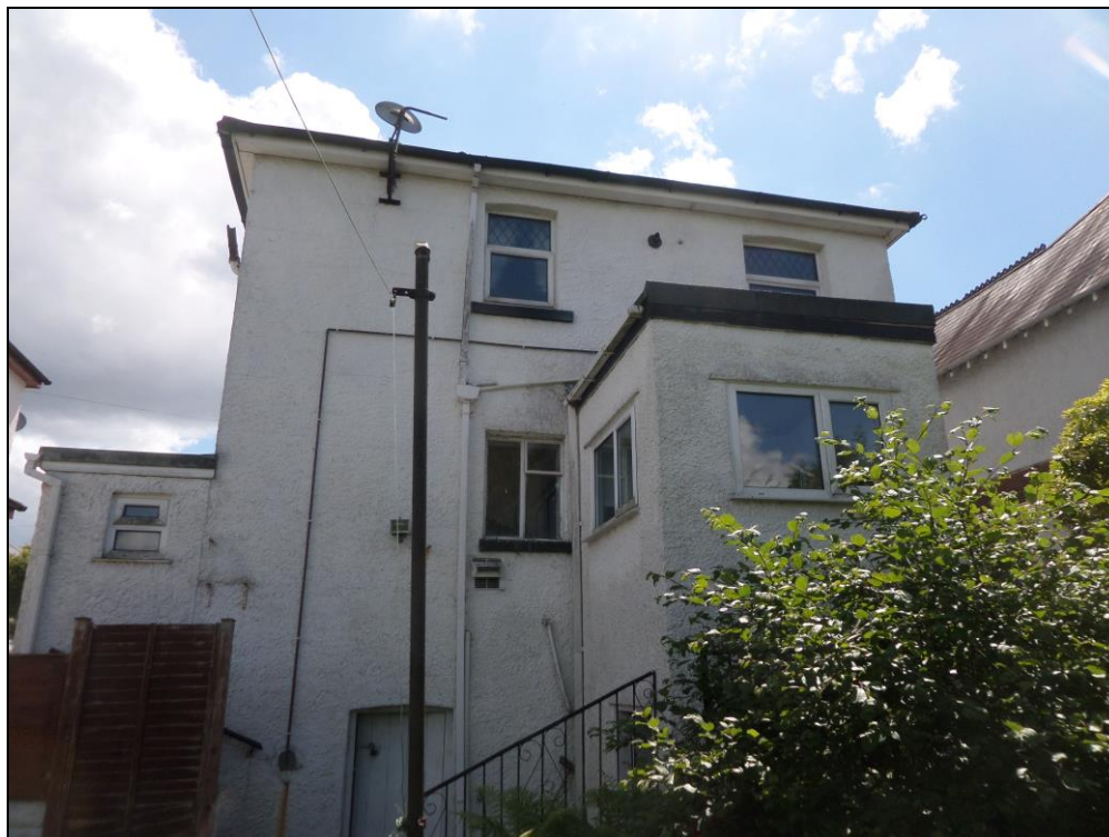
Photo 3: Three storey northern elevation (view looking south).
