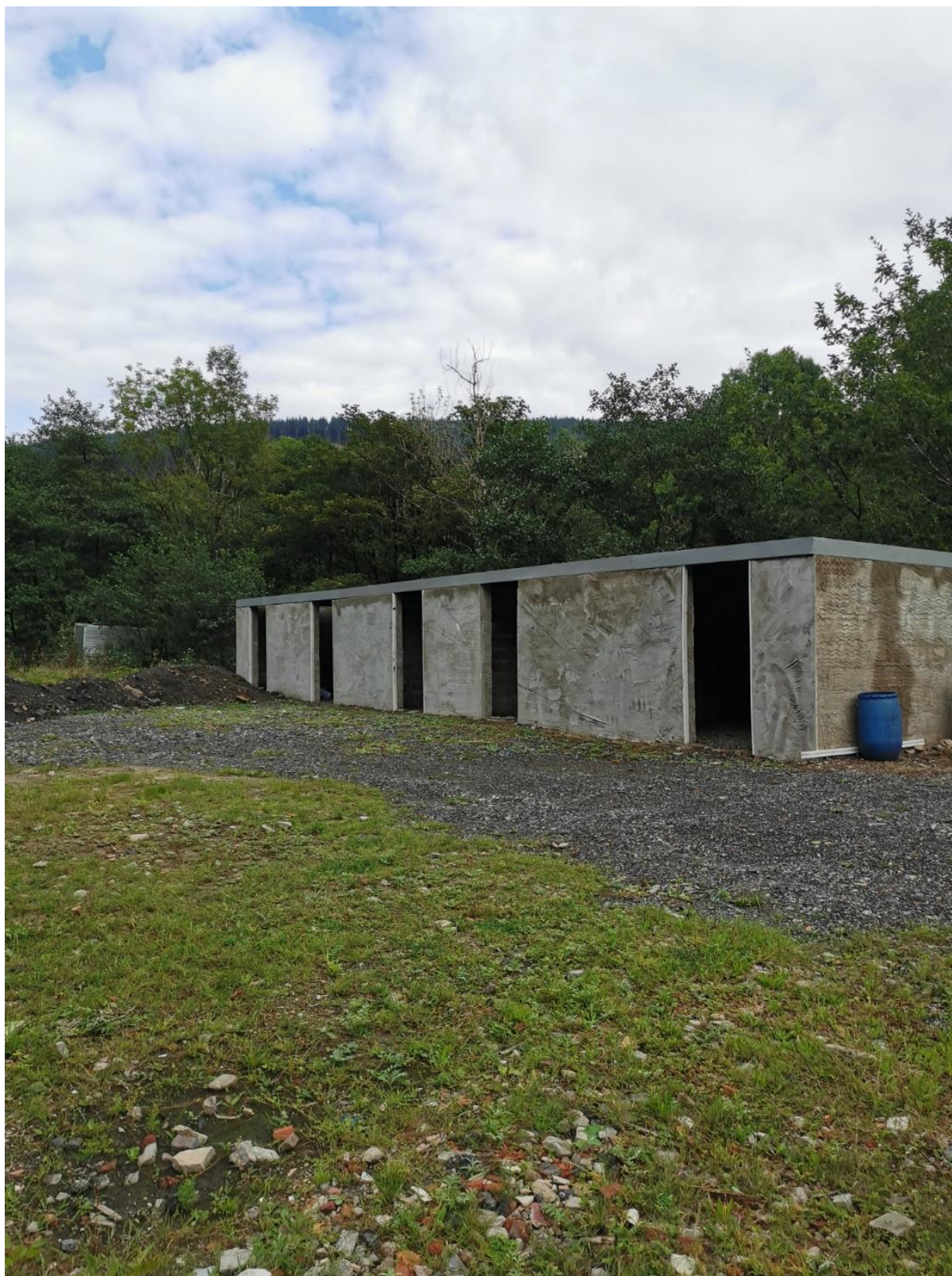
Plate 2: Existing stable block.
