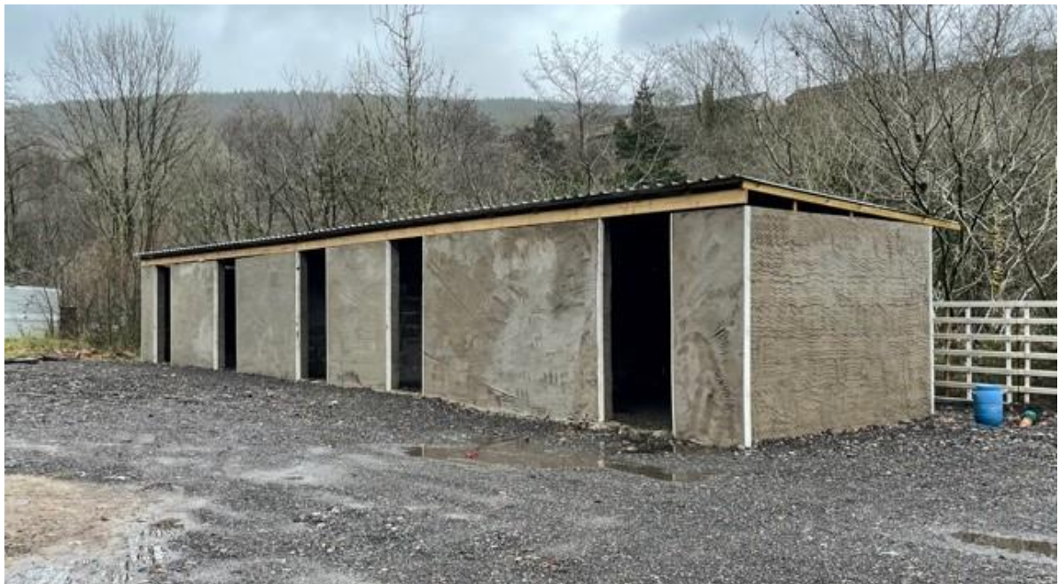
Photograph showing the block of stables and small storage shed
