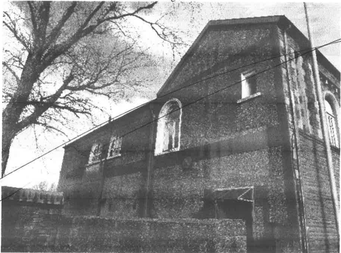
Photo 25 – Left Side Wall Elevation (Upper)
