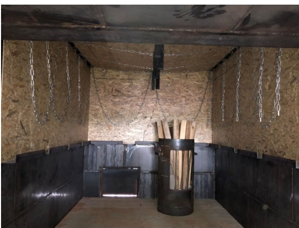
Correct placement of the wood in the fire room
