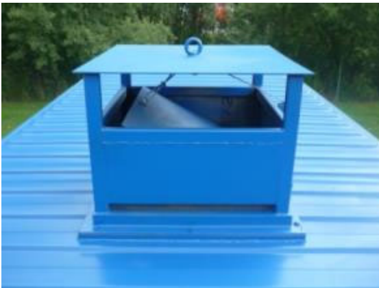
Chimney with lockable flap on the roof of the observation room covered by a special rollover extraction hood (hood made of stainless steel)
