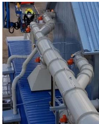
Chimney with lockable flap on the roof of the observation room covered by a special rollover extraction hood (hood made of stainless steel)
