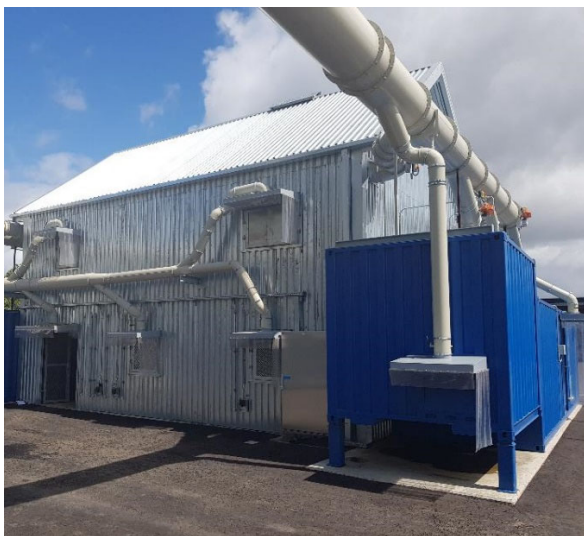
Building structure with demo/attack unit
