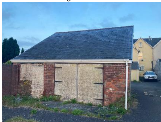
Photo 10: West facing rear of Rear Extension
