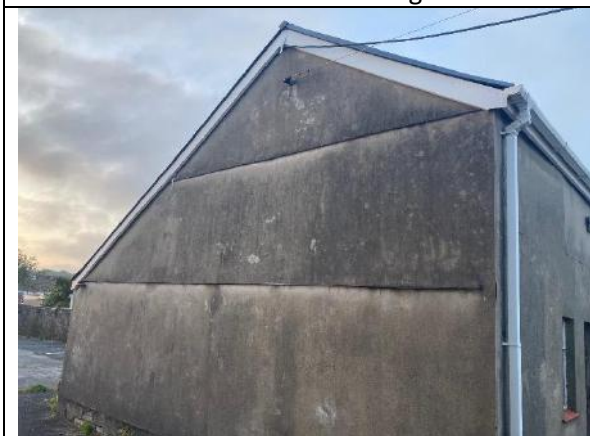
Photo 9: South facing side of Rear Extension
