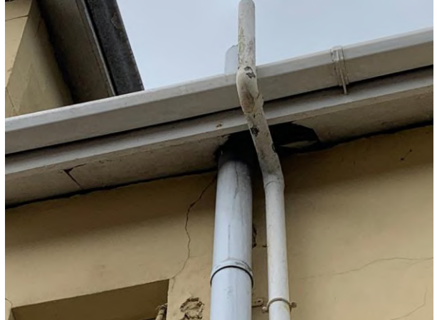
Photo 18: Hole in Soffit of Extension on the North-Eastern Elevation
