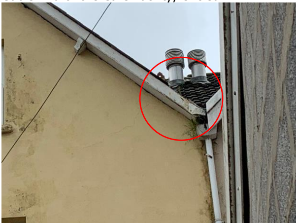
Photo 11: Missing Slate on the North-Western Gable End of the Care Facility, Circled
