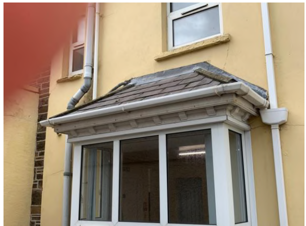
Photo 12: Lead Flashing on the Dormer Window
