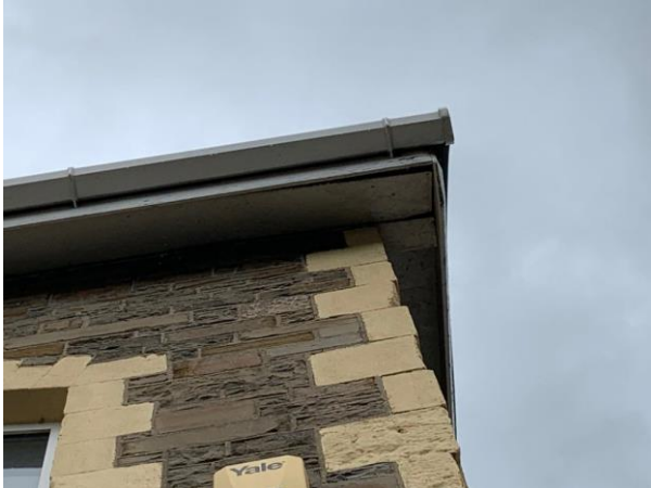
Photo 17: Gap in Timber Soffit of Extension on the North-Western Elevation
