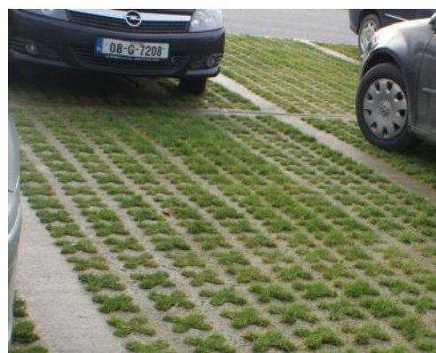
Figure 11 Grasscrete used and accepted widely for vehicle parking and as a surface drainage system
