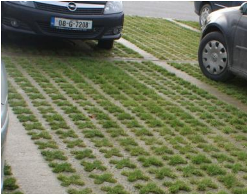
Figure 11 Grasscrete used and accepted widely for vehicle parking and as a surface drainage system
