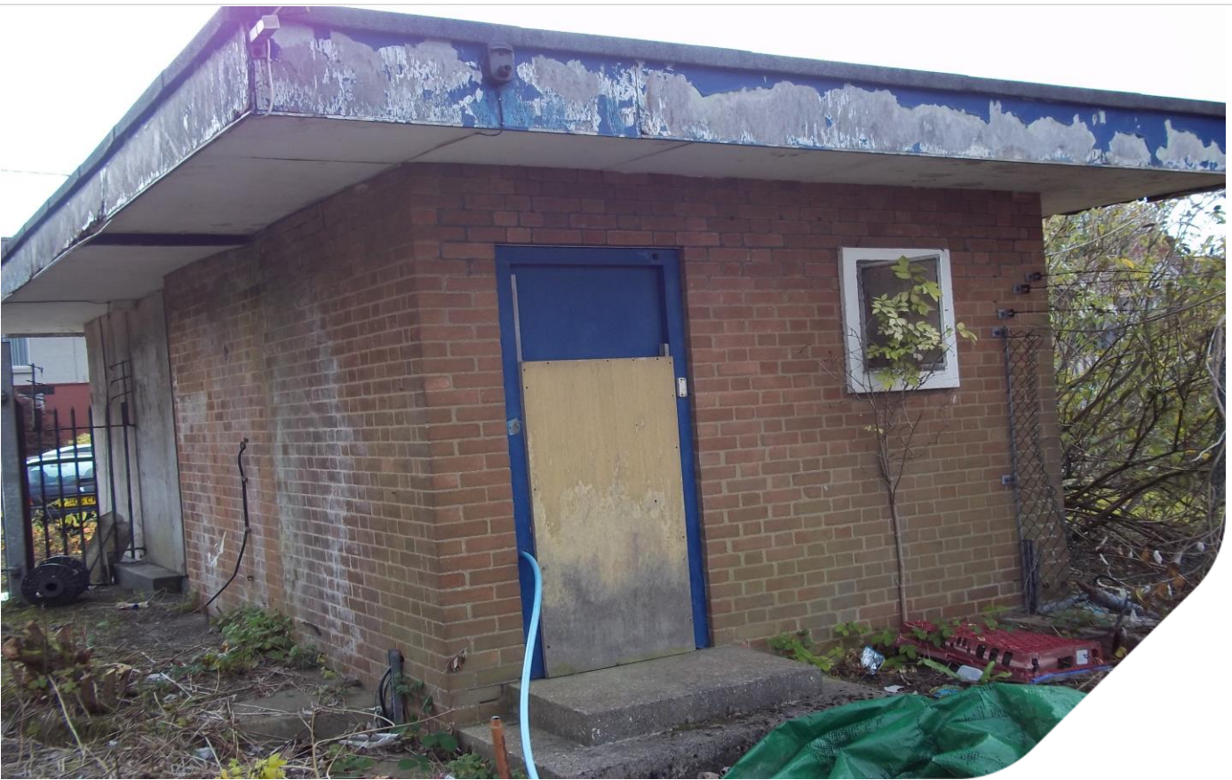
Plate 11: Gatehouse at southern entrance..
