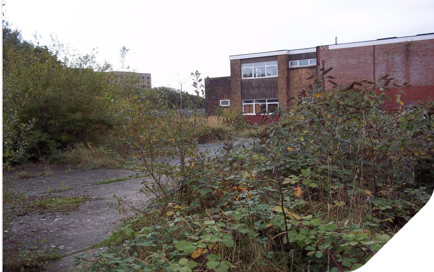
Plate 05: Concrete slab looking southwest.
