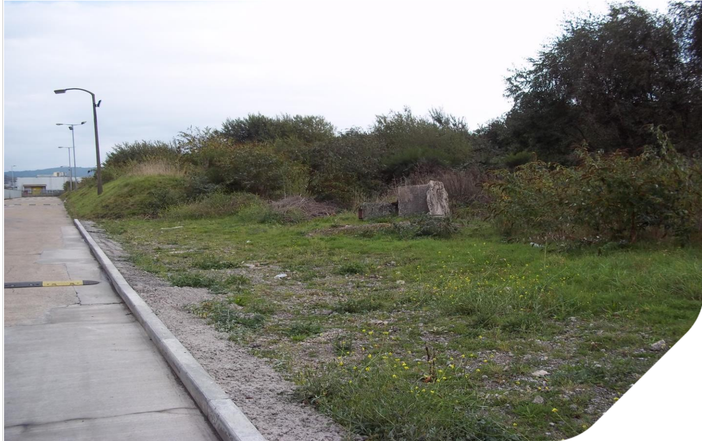
Plate 01: Northern perimeter bund looking east and masonry debris.
