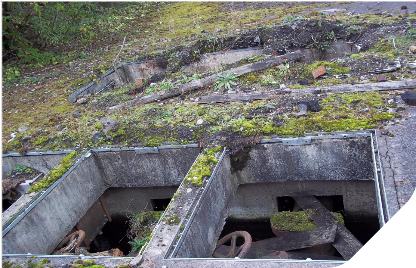
Plate 10: Car park interceptor drainage southern perimeter.
