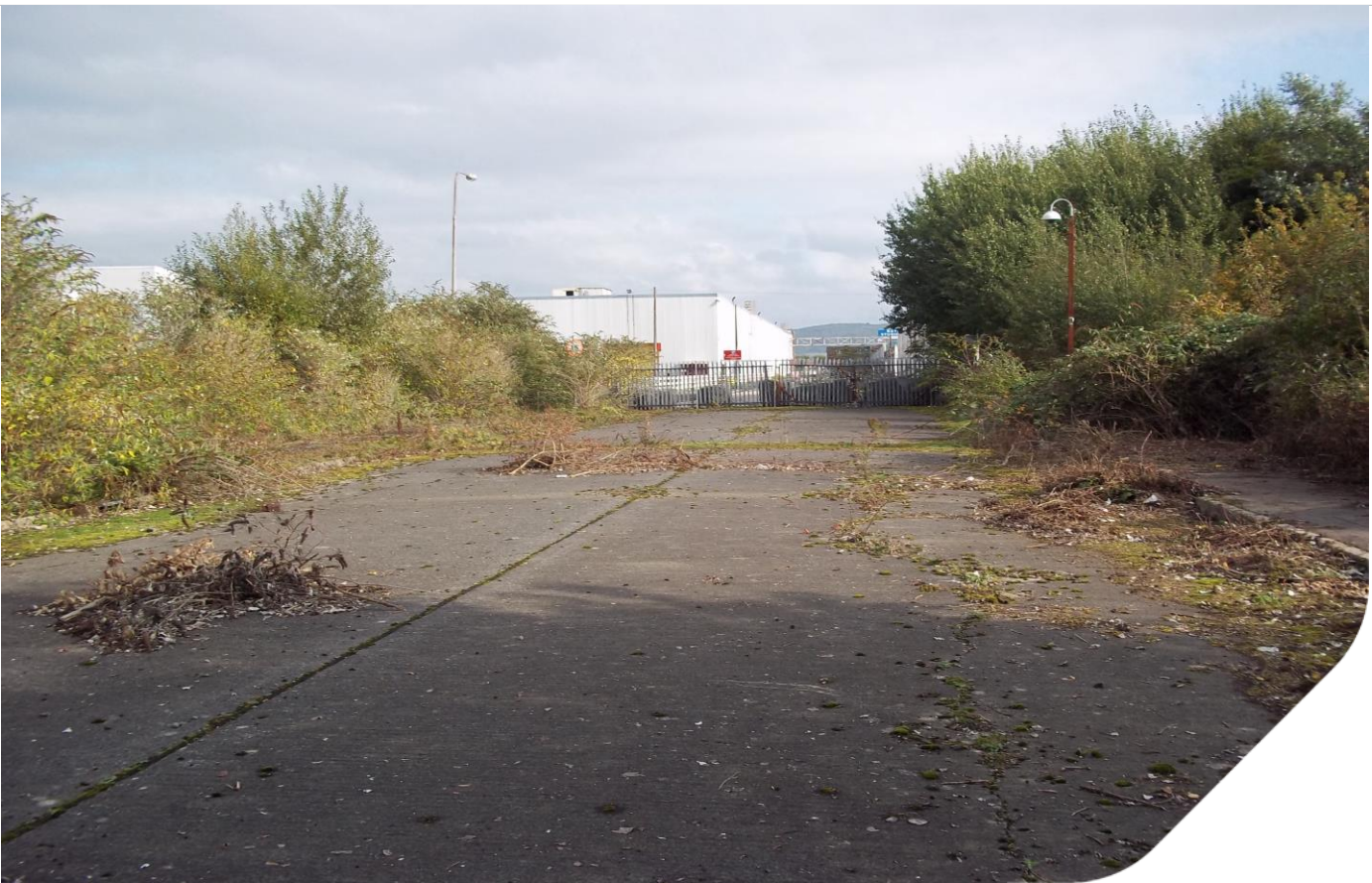
Plate 04: Concrete road looking east_____
